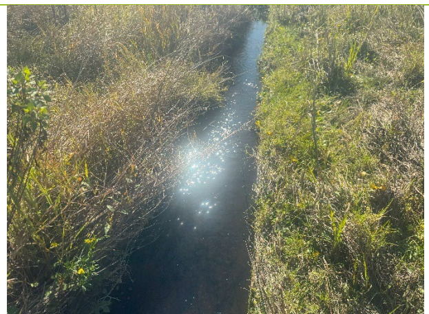
Photo plate 6: drainage channel
