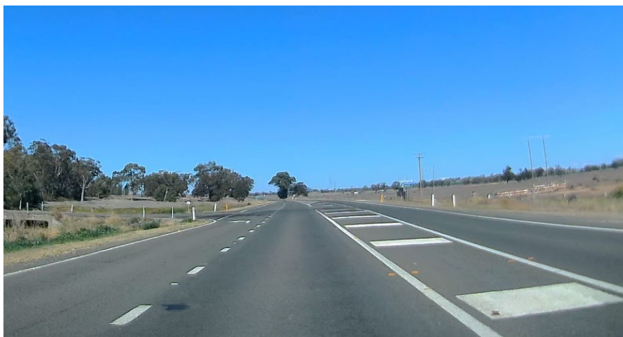
Figure 3.3: Kamilaroi Highway at Rangari Road
