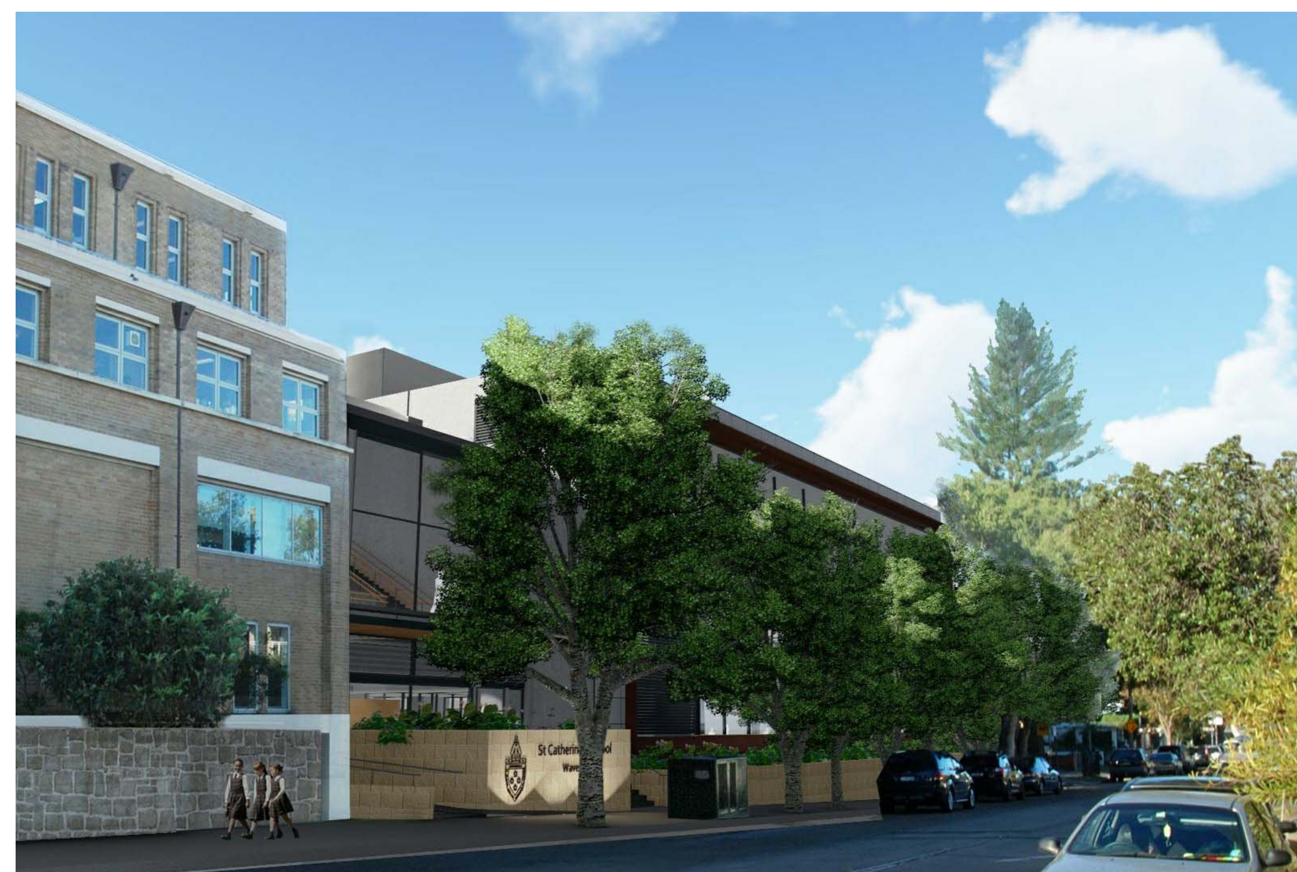
VIEW 2 - LOOKING NORTH EAST FROM MACPHERSON STREET - (S.96)
