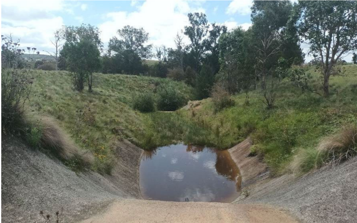
Figure 7.12 Concrete spillway and associated earthworks in SU2, view northwest.
