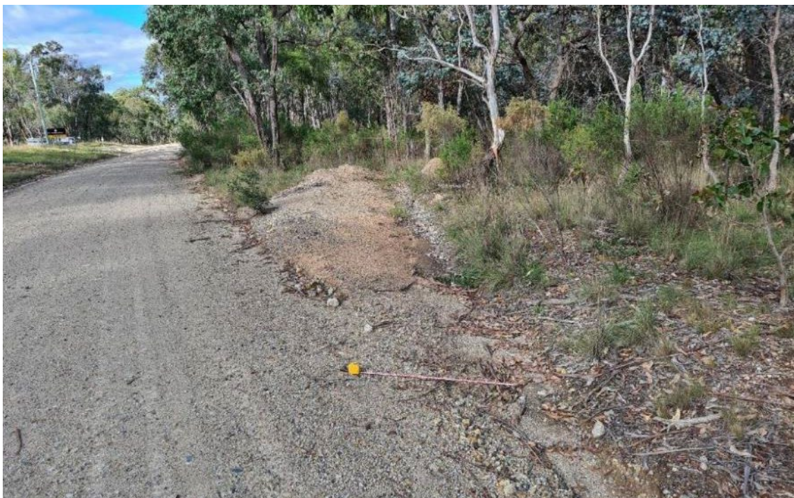
Figure 7.33 Disturbances from table drain, GSV and exposures on road shoulder in SU9, view east.
