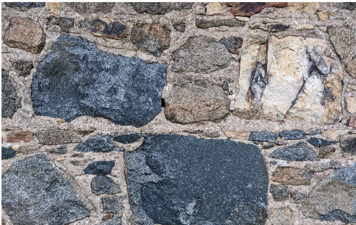
Figure 2.10 Stonework detail on Arthursleigh woolshed.
