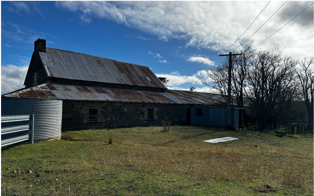
Figure 1.24 North-facing view of Arthursleigh woolshed.
