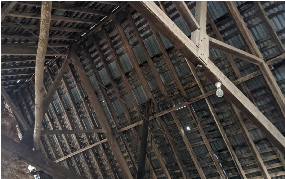
Figure 1.21 Interior detail of Arthursleigh woolshed.
