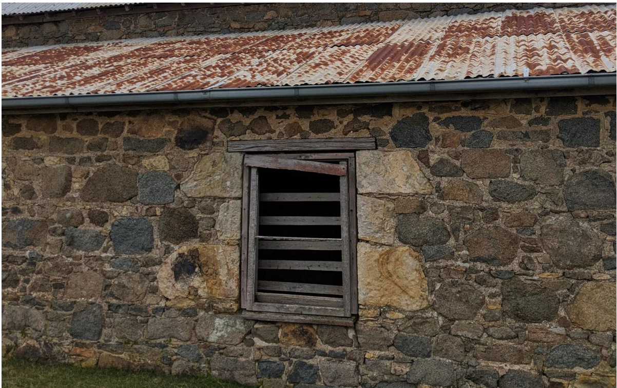
Figure 1.19 North-west facing view of the Arthursleigh woolshed.
