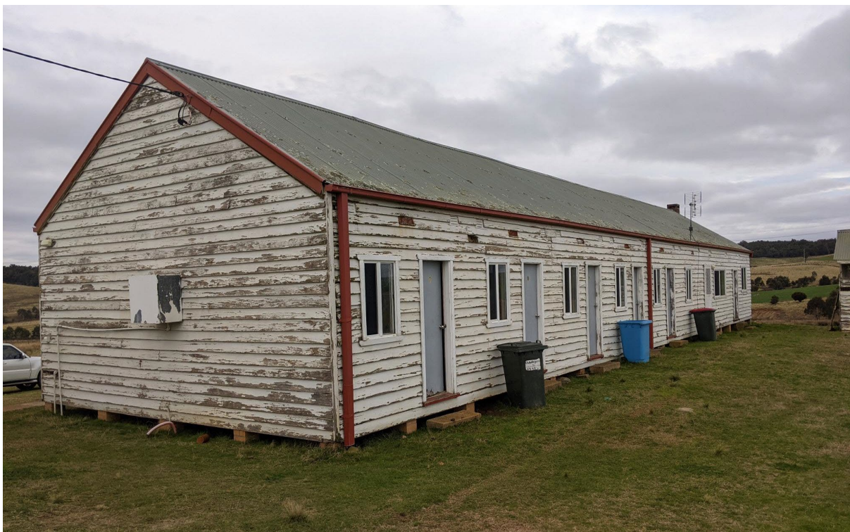
Figure 1.27 North-east facing view of the Arthursleigh shearer's quarters.
