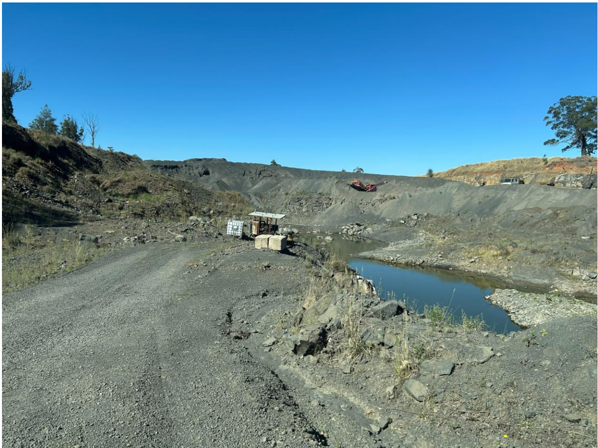
Photo 12: Main quarry sump with transfer pump. IBC adjacent to the pump is empty and awaiting removal.
