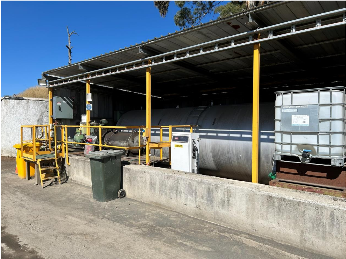
Photo 5: Main liquid store. Roof in good condition.
