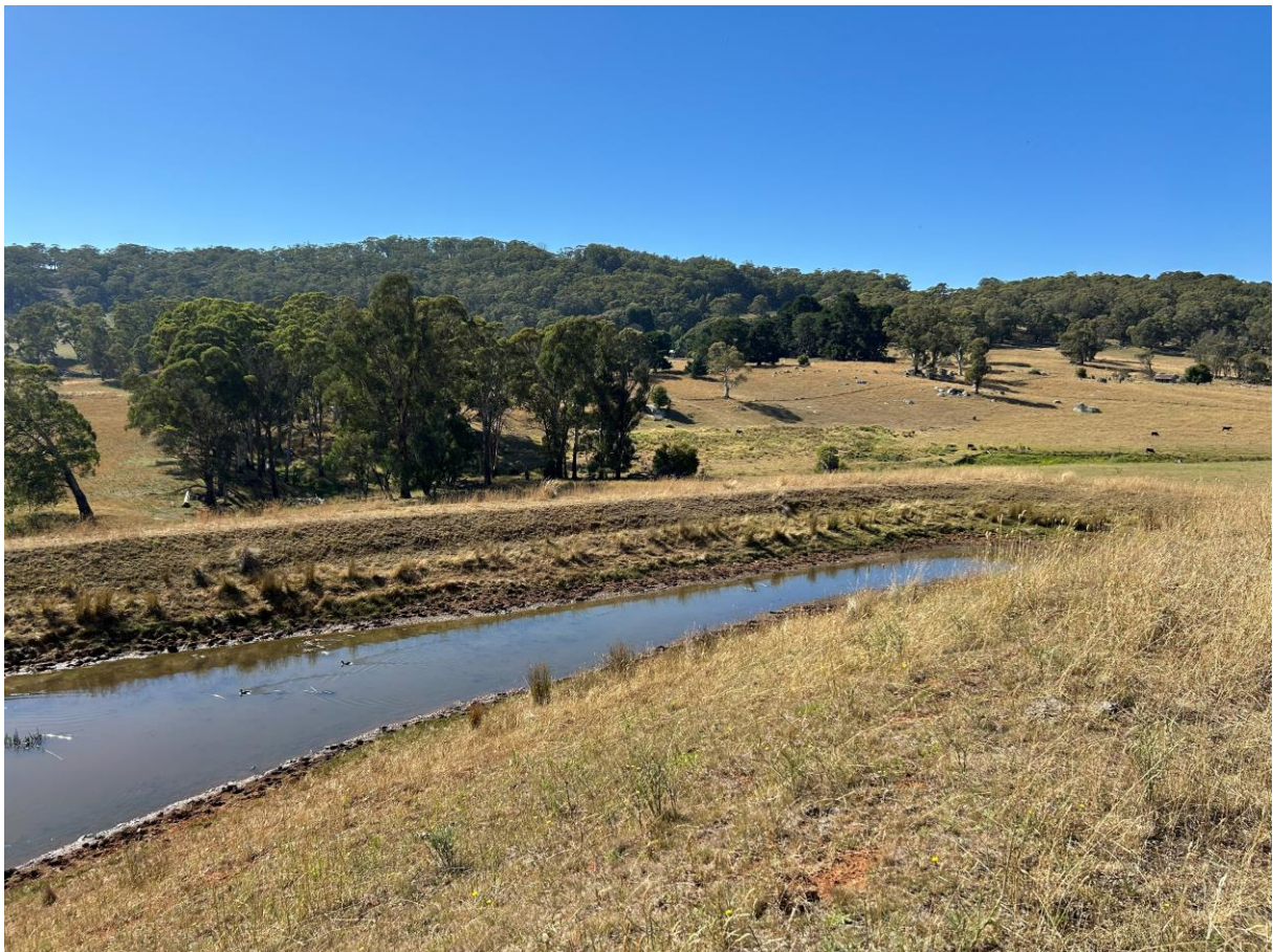
Photo 10: Lower of three sediment dams, showing significant freeboard.
