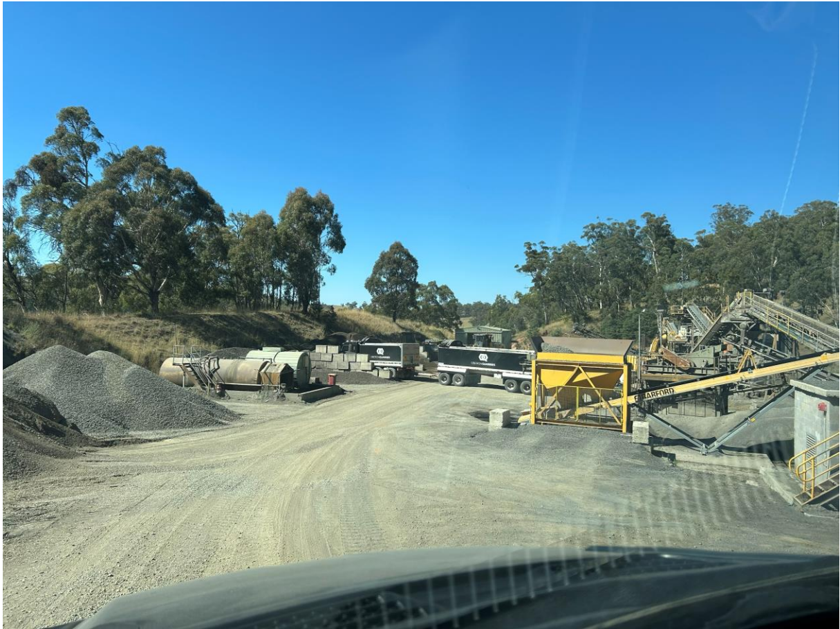
Photo 21: Crushing plant area. Secondary liquid store for pre-coat aggregate on the left of the image.
