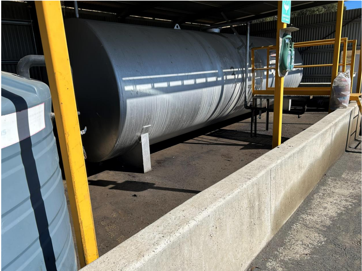
Photo 7: Main liquid store, showing bunding condition. Minor staining on outside of concrete – no staining on gravel surfaces or elsewhere. Staining appears to be historic and not due to any notable accumulation of liquid in the bund, drips etc.
