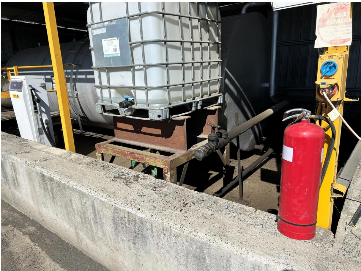
Photo 6: Main liquid store, showing bunding condition. No accumulated liquid in bund.
