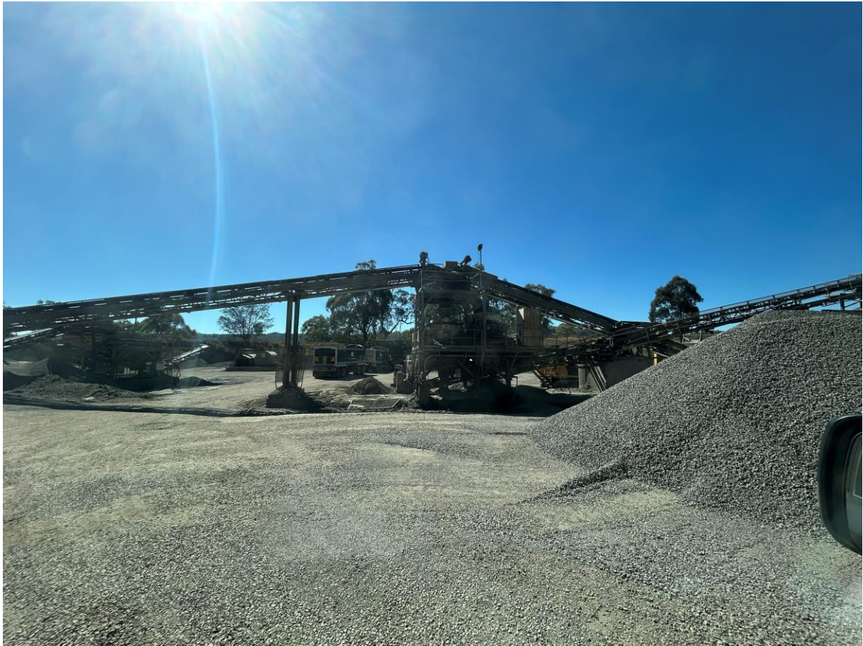
Photo 23: Crushing train and 10mm aggregate stockpile in foreground.
