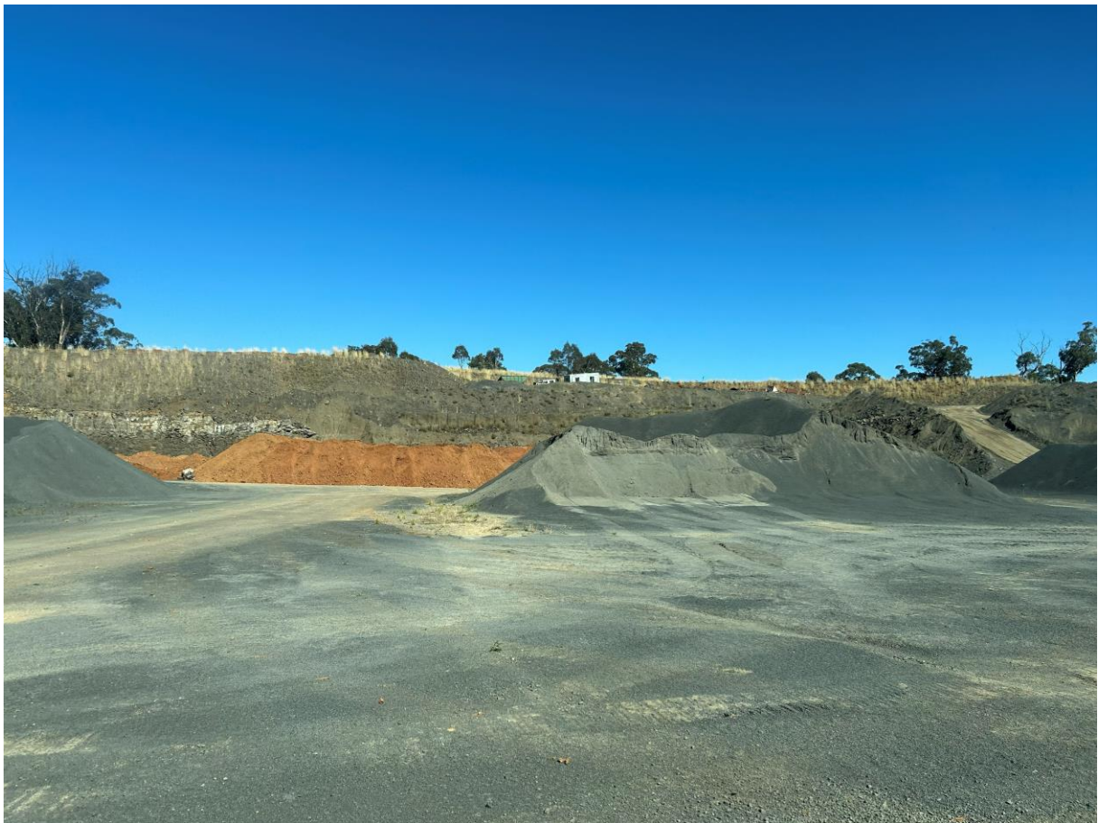
Photo 18: Northern part of the pit. Crusher dust in the foreground and residual clay topsoil stockpile in the background.
