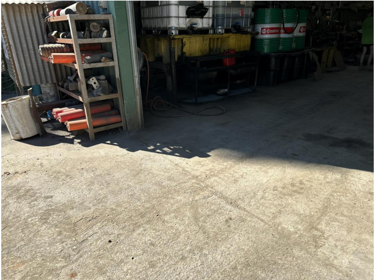
Photo 29: Door leading to workshop showing very minimal staining and absence of any drips or evidence of hydrocarbon/liquid chemical escape from workshop.
