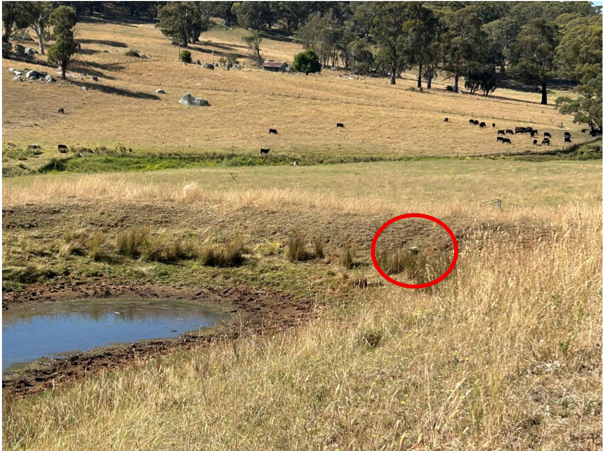
Photo 11: Lower of three sediment dams, showing outlet (discharge) pipe (in red) and significant freeboard.
