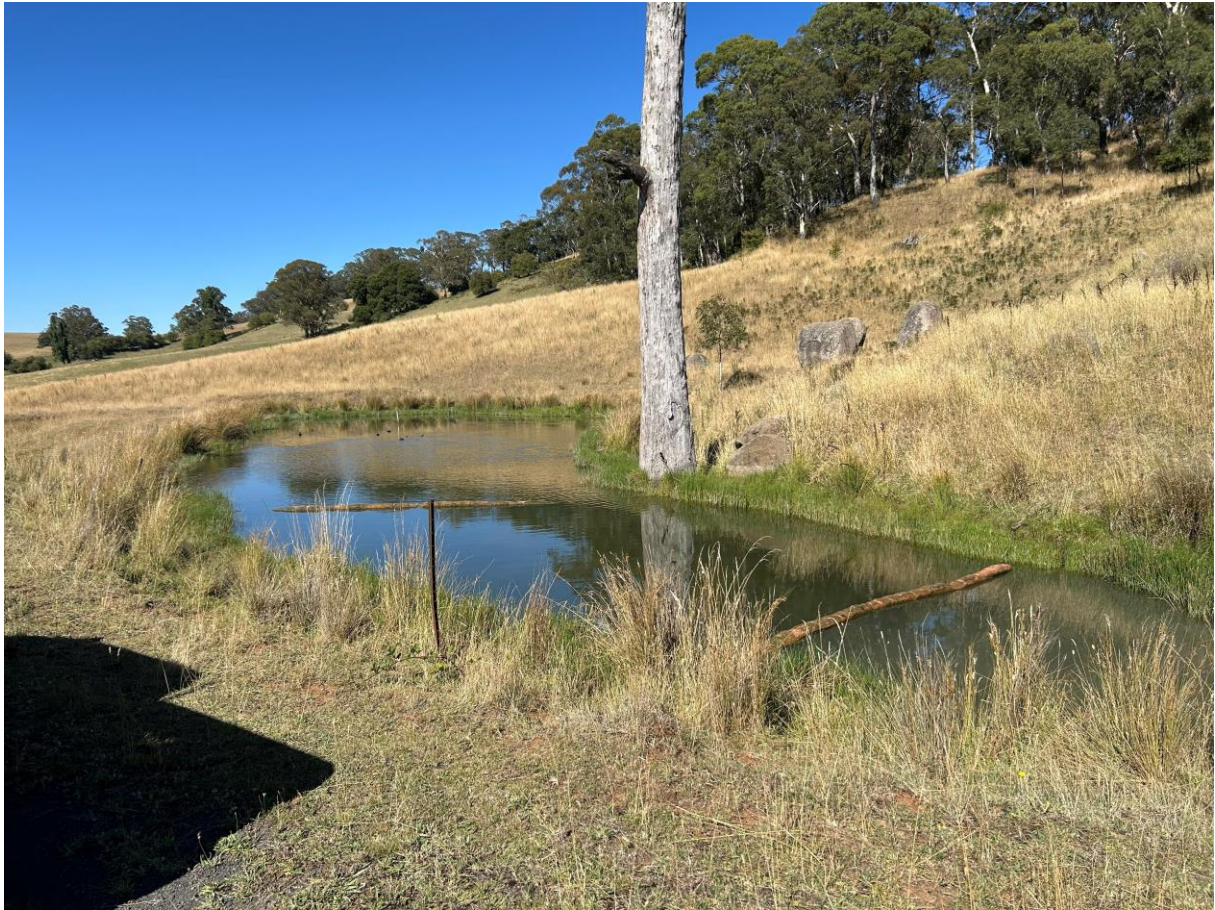
Photo 9: Upper of the series of three sediment dams for the Site. These dams capture run off from the office and roadway area. The pit and exposed extraction areas all drain to the quarry void.
