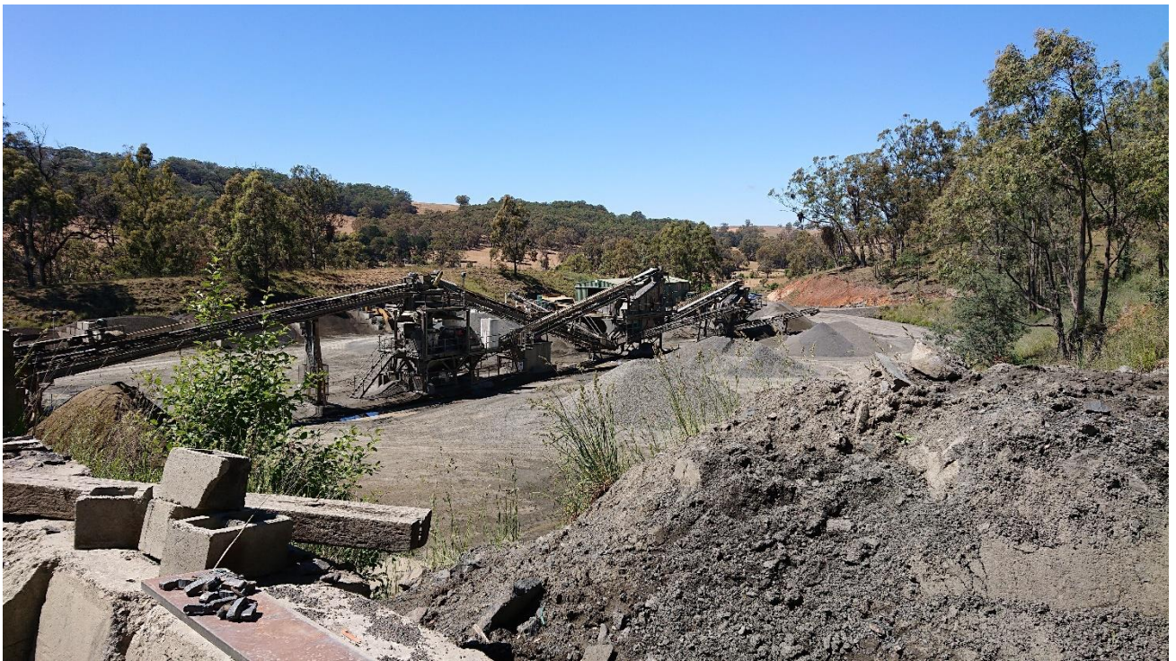
Photo # 1 - Crusher Plant
