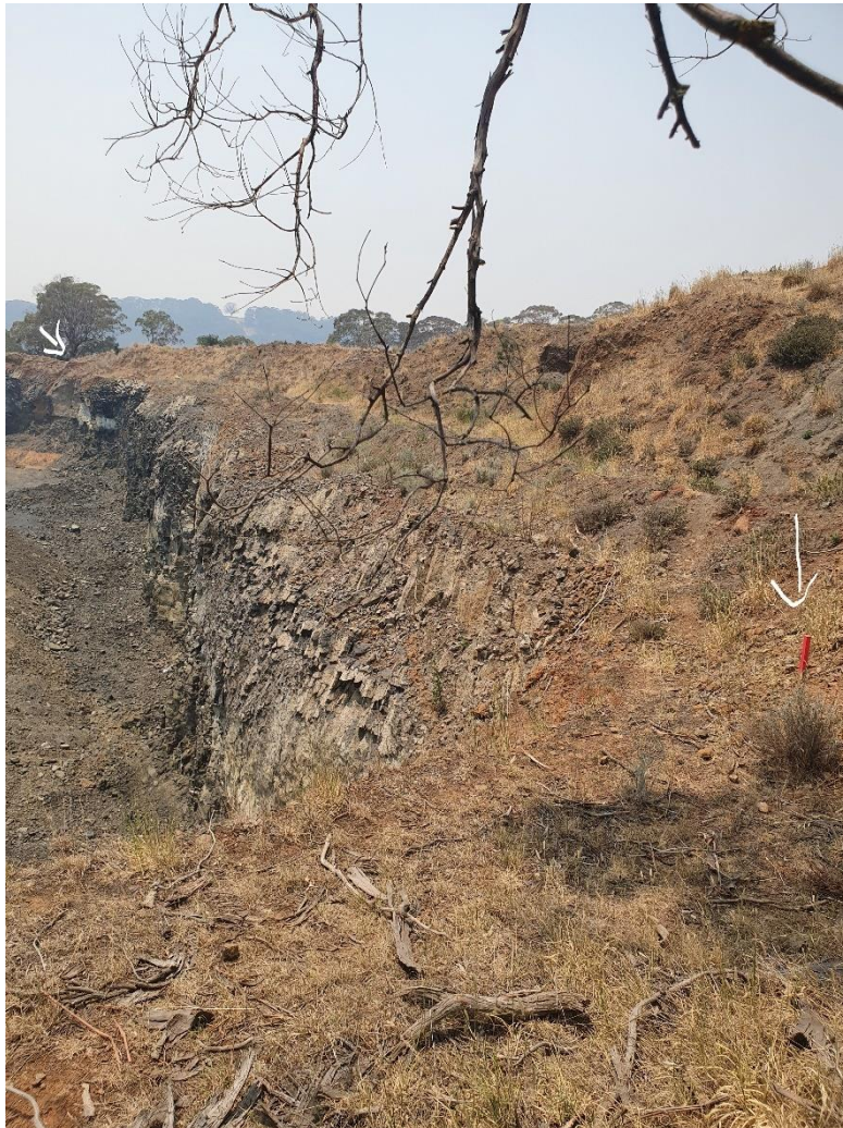
Photo # 8 - Limit of Excavation Markers
