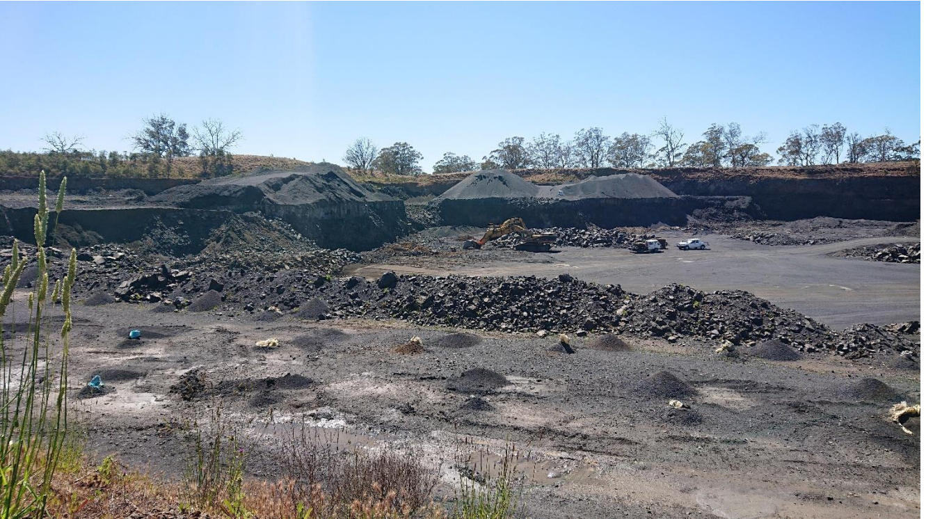
Photo # 2 - Quarry Pit
