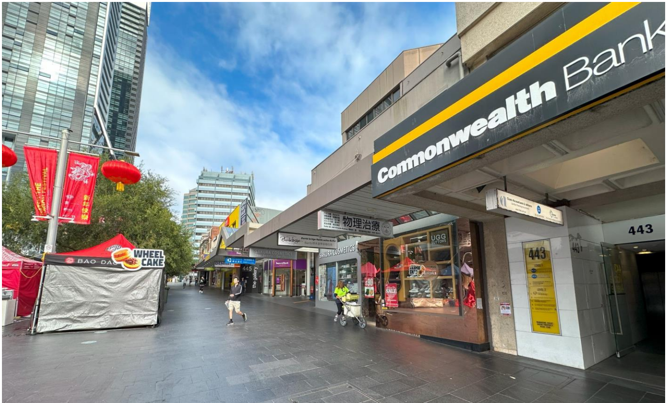
Figure 12 Existing Built Form on the Northern Side of Victoria Avenue (to the north of the Site)
