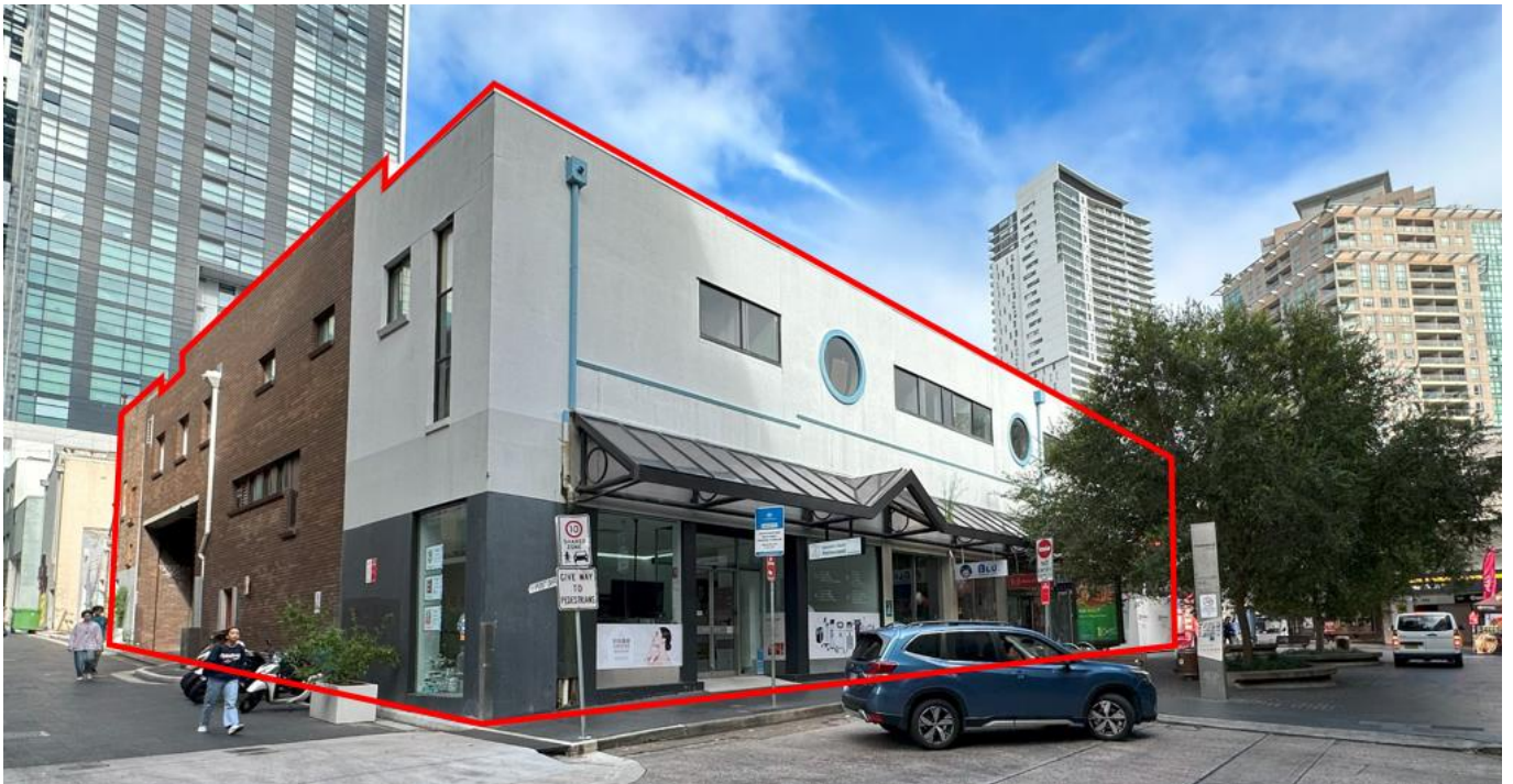
Figure 6 Existing Development to Victor Street Frontage (looking north-west, subject Site outlined red)
