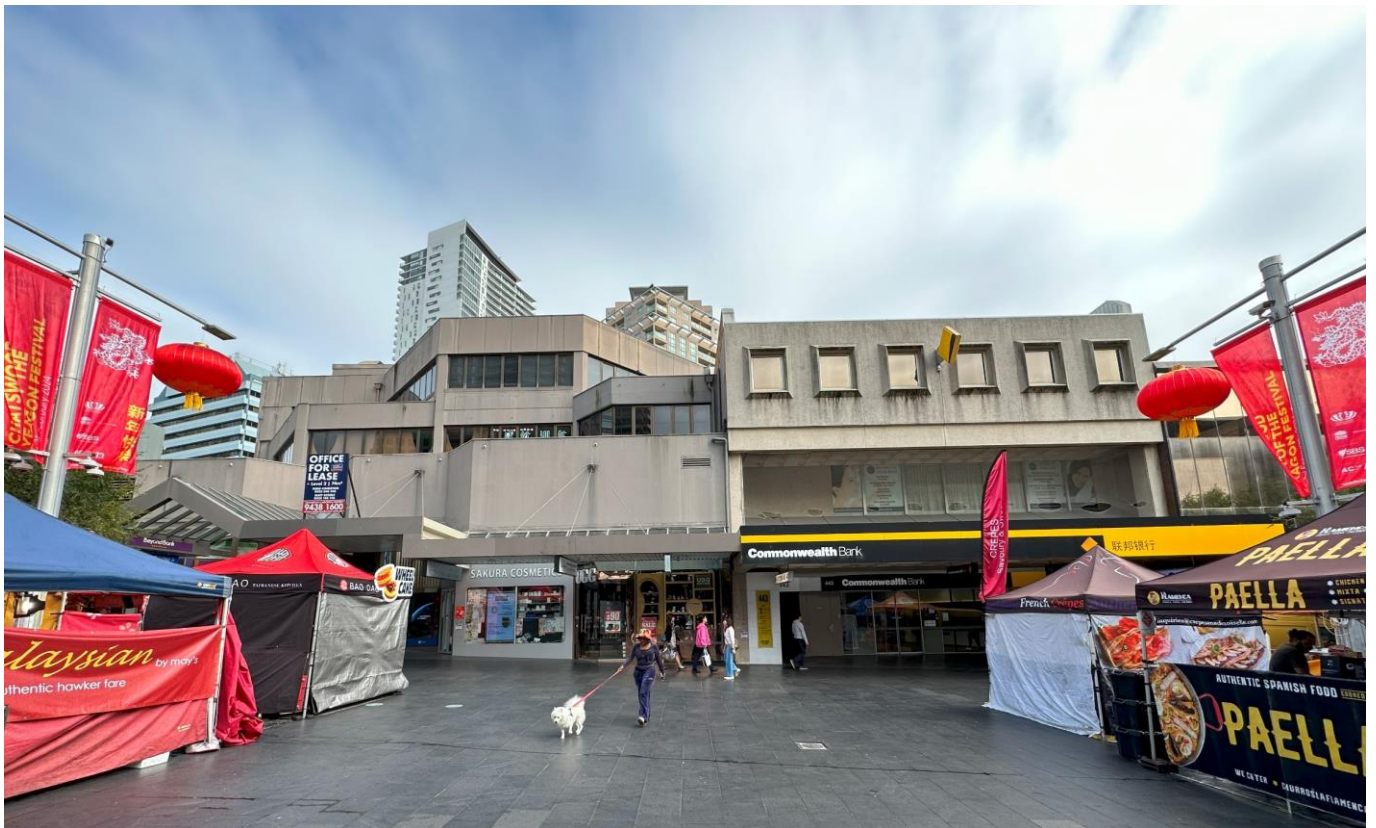
Figure 13 Existing Built Form on the Northern Side of Victoria Avenue (to the north of the Site)
