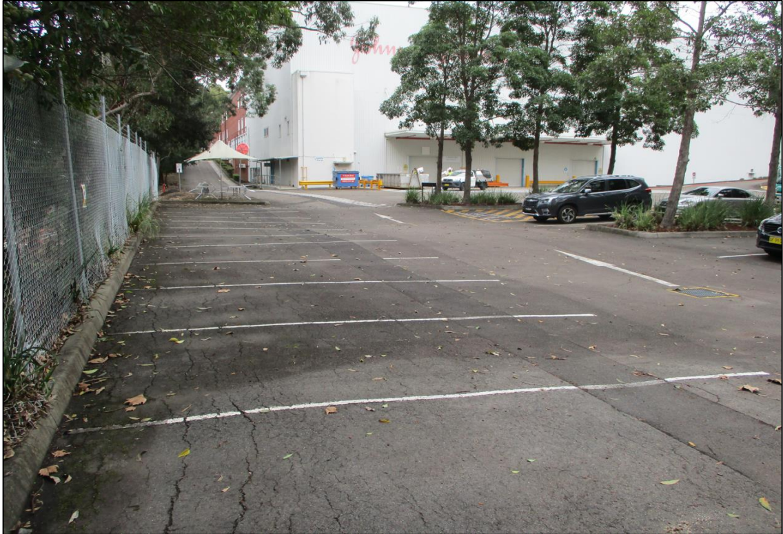
Photo 1: South western end of site, asphalt car park on-grade.
