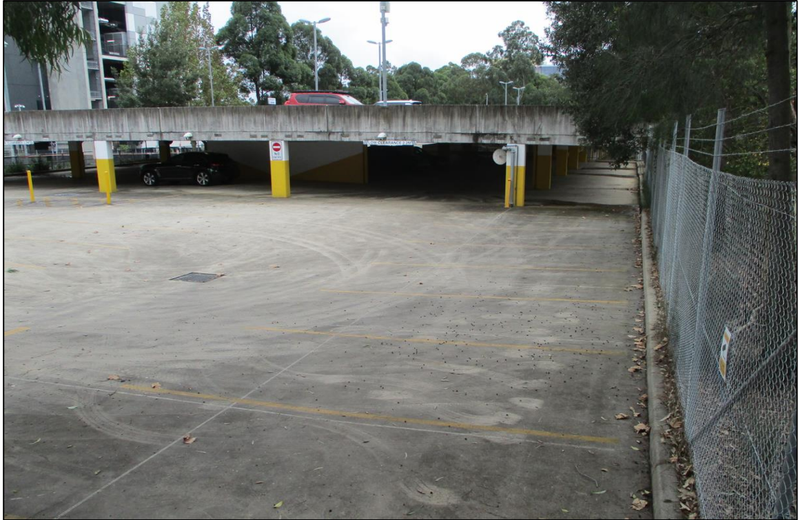
Photo 3: Central part of site, concrete carpark structure.
