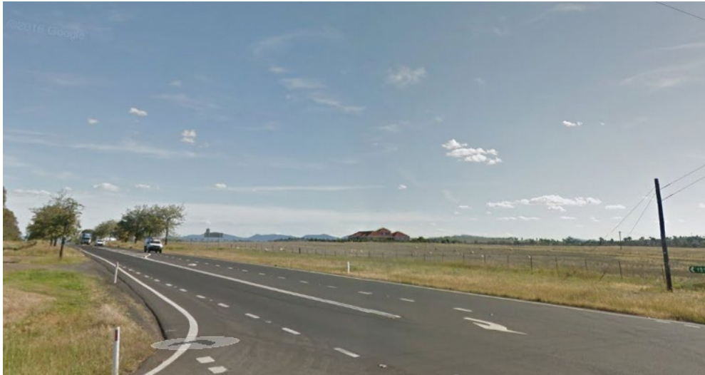
Figure 4-8: New England Highway facing south at Burgmanns Lane
