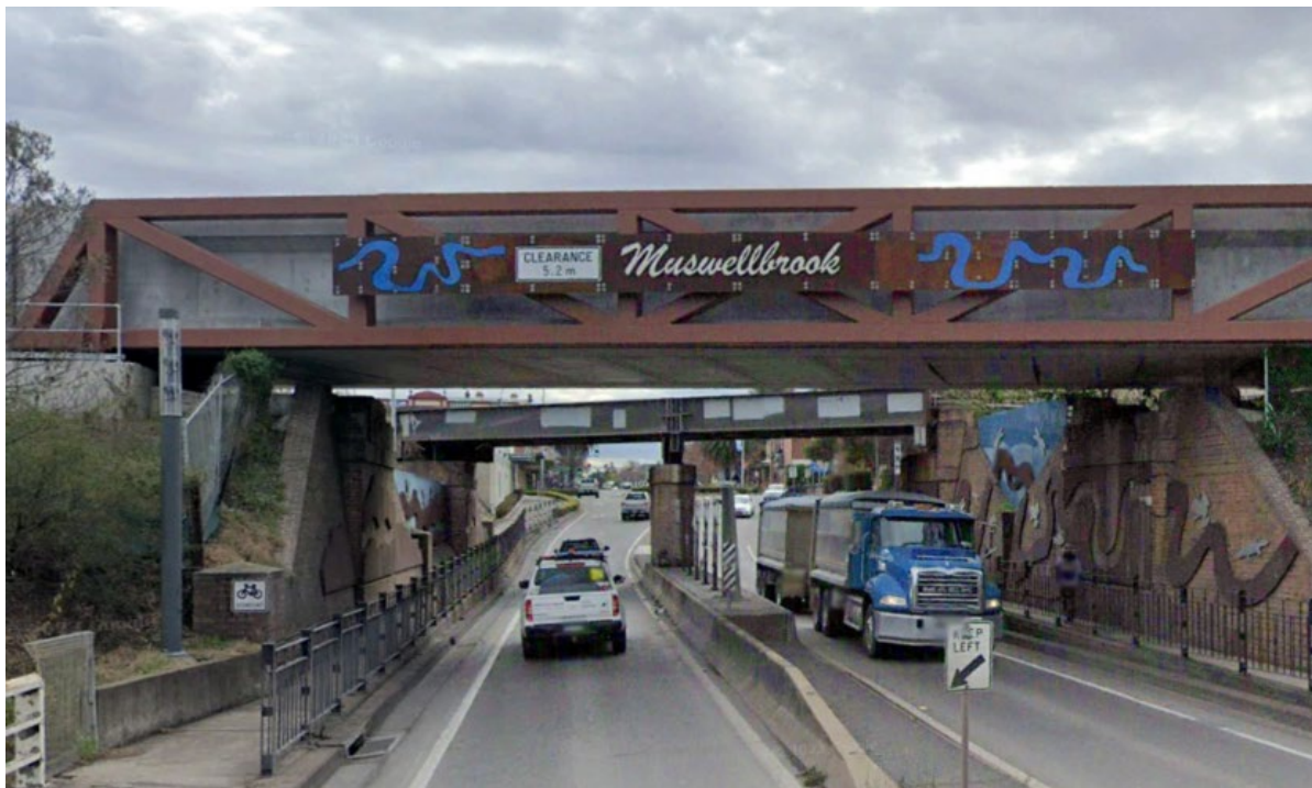
Figure 4-3: 5.2 metres height restriction under railway overbridge on Sydney Street, Muswellbrook
