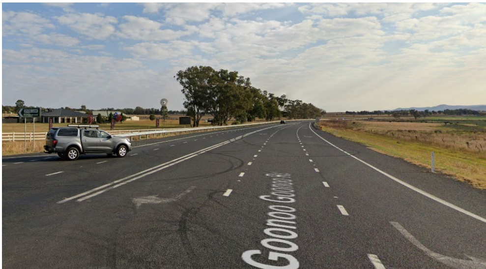
Figure 4-9: New England Highway facing north at Whitehouse Lane
