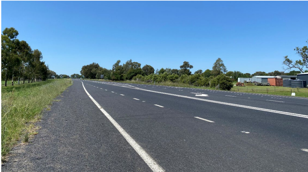
Figure 4-10: New England Highway facing south at Whitehouse Lane
