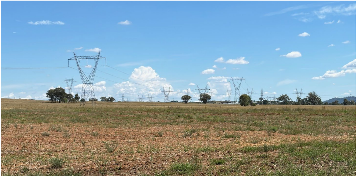
Figure A-2: Example of steel lattice structure (currently present on the Project Site)
