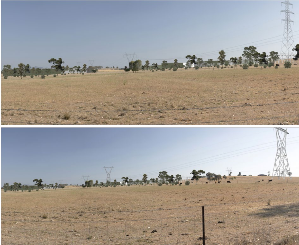
Figure A-3: Illustration of Project from Burgmanns Lane highlighting existing transmission infrastructure and proposed screening vegetation, noise walls, ancillary infrastructure, BESS substation and transmission tower (Solution 1 = top, Solution 3 = bottom)
