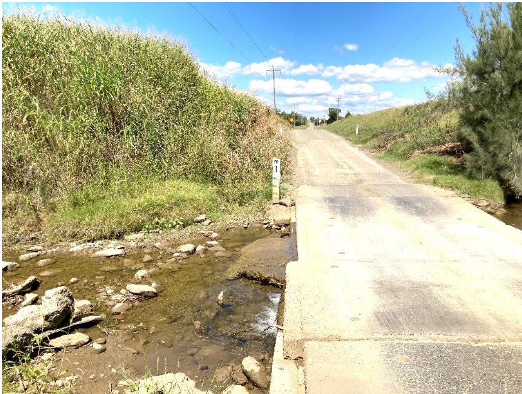
Figure B-10: Burgmanns Lane at Goonoo Goonoo Ck - looking east
