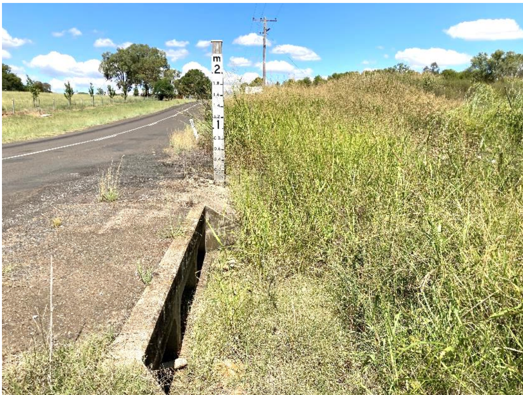
Figure B-12: Whitehouse Lane at Goonoo Goonoo Ck box culverts - looking east
