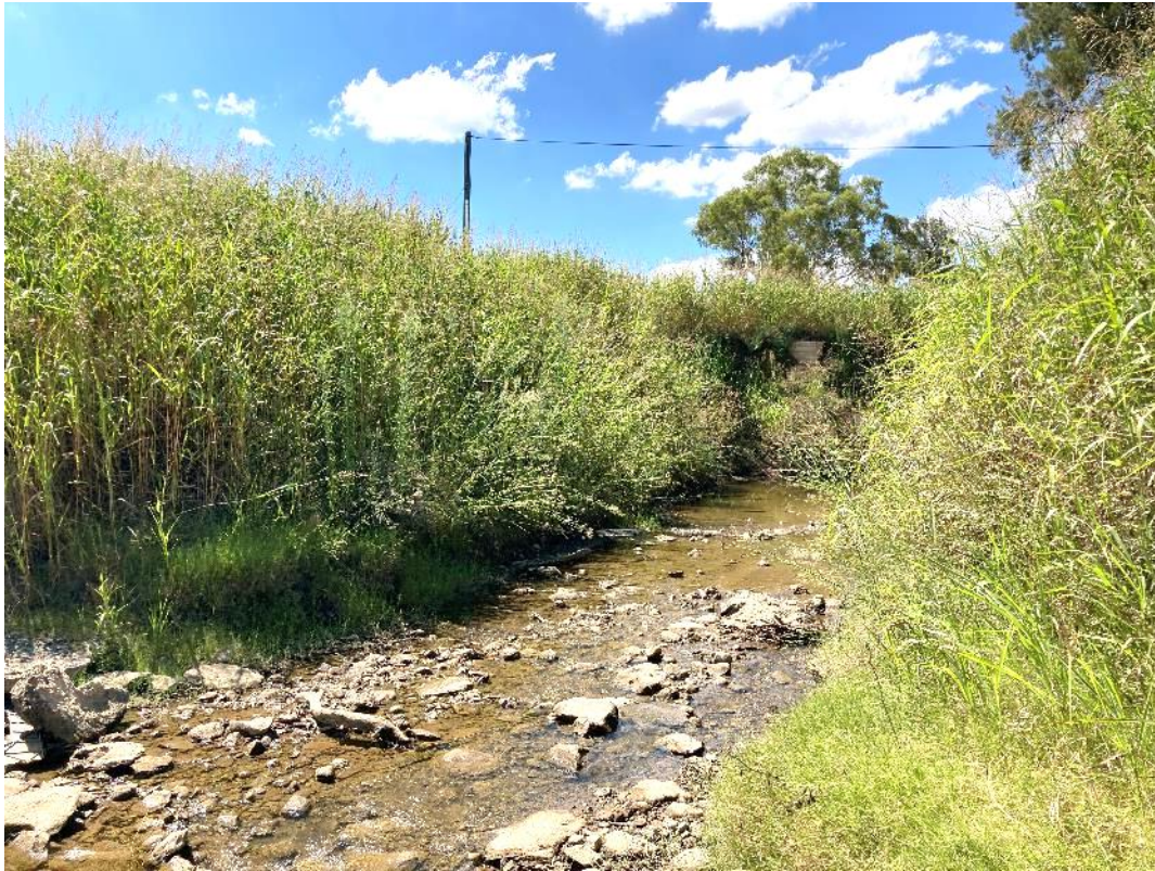
Figure B-9: Burgmanns Lane at Goonoo Goonoo Ck - looking north
