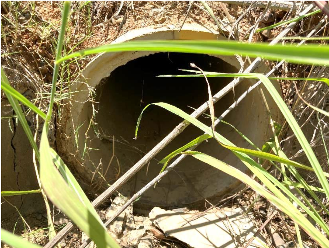
Figure B-5: Ascot-Calala Rd at Burgmanns Lane – cross drainage culvert (approx. 450mm diameter)
