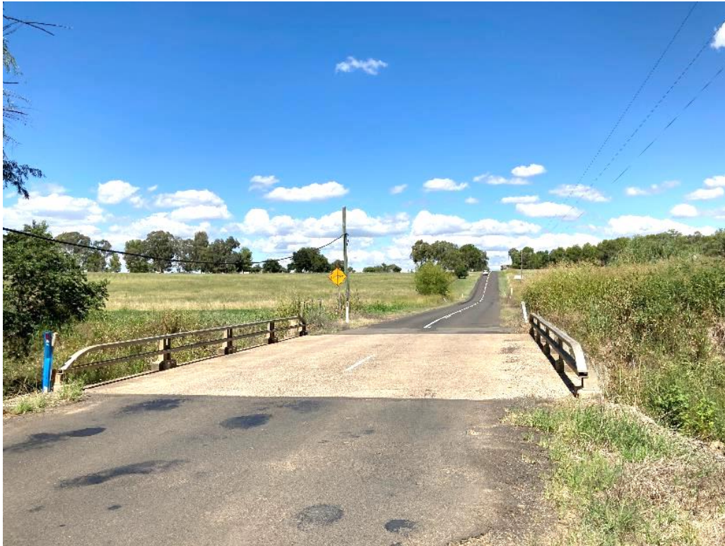
Figure B-13: Whitehouse Lane at Goonoo Goonoo Ck bridge - looking east
