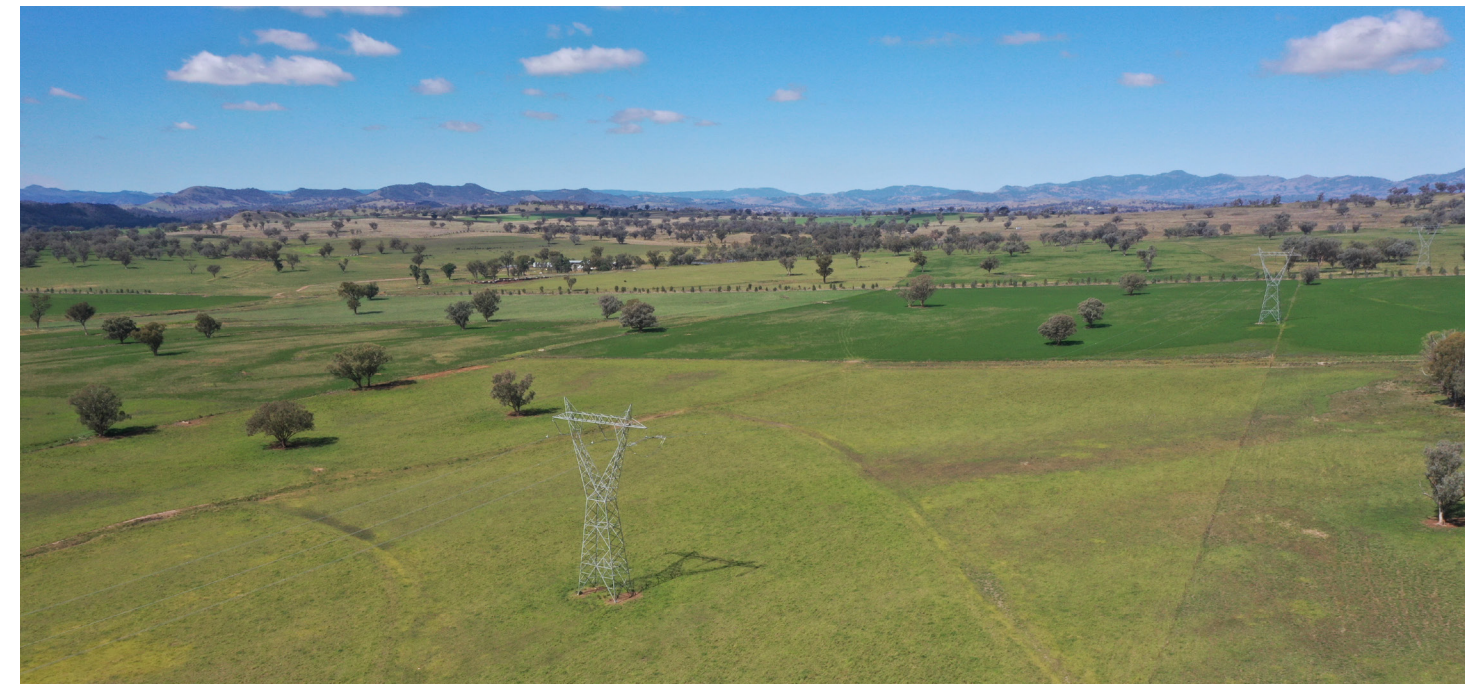
Image 04 – (Drone Image) Agricultural Pastures with Transmission Lines Above (Moir LA - 04/2023)
