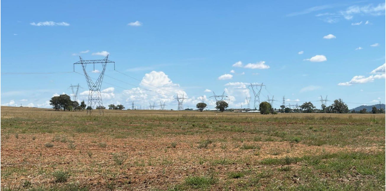
Figure 3-2 Example of steel lattice structure (currently present on the Project Site).
