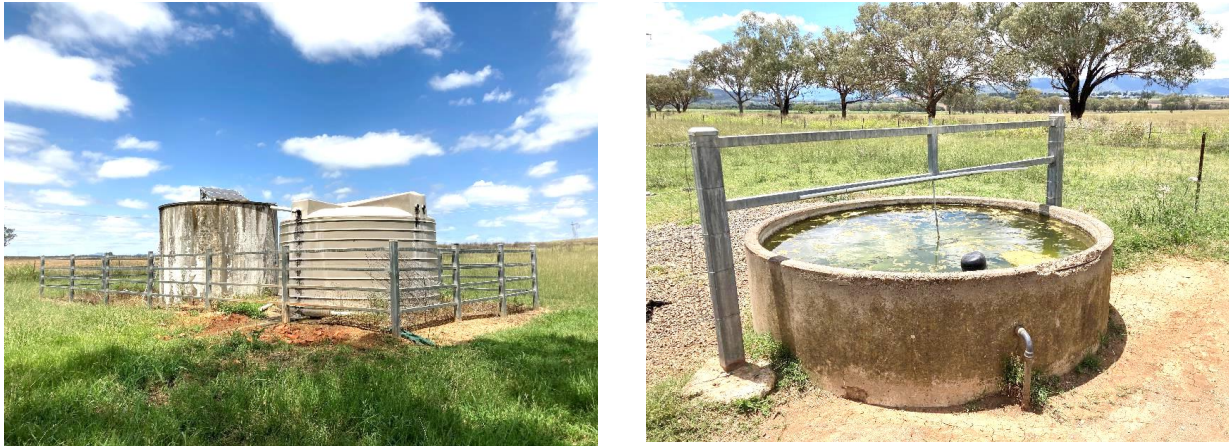
Figure 6-19 Existing groundwater bores within the Project Site (left - GW055998, right - no known ID)
