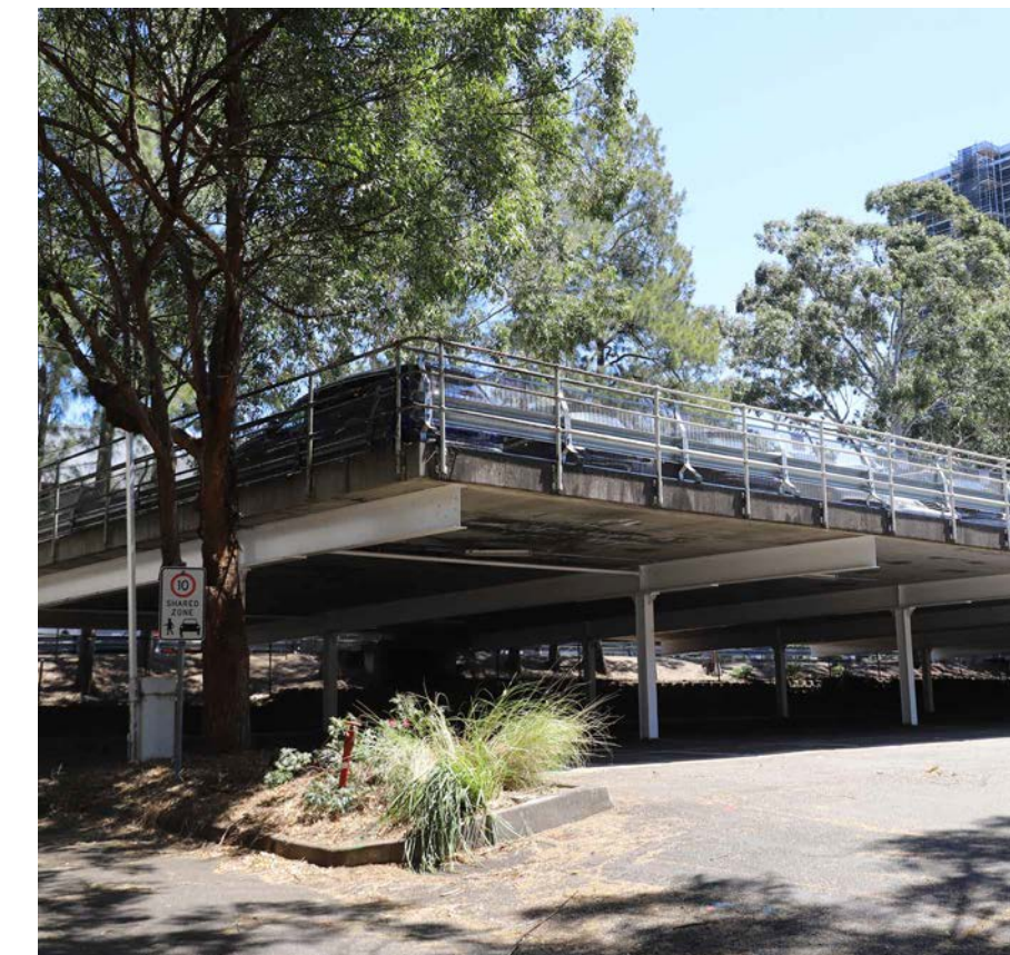
Photo 7. Elevated car park within the site.
