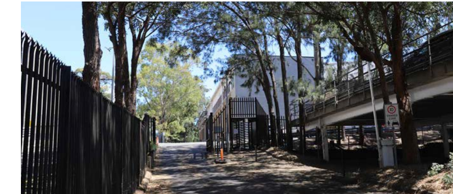
Photo 8. South-west view along internal site road.
