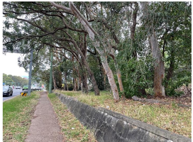
Picture 6 Footpath along Lane Cove Road
