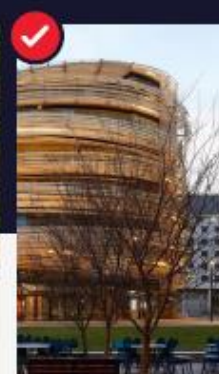
Landmark Gateway Building
