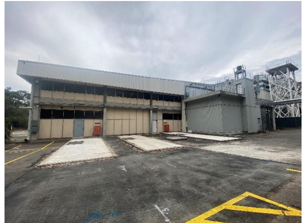
Figure 9 – Views towards warehouse 2 from the rear of the subject site, looking northeast.
