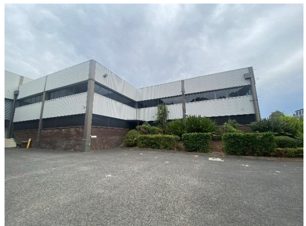
Figure 7 – Views west towards warehouse 1.
