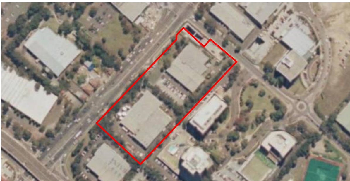
Figure 18 c.2004 aerial image of the subject site within the context of its immediate locality. The extant subject boundary curtilage is outline in red.
