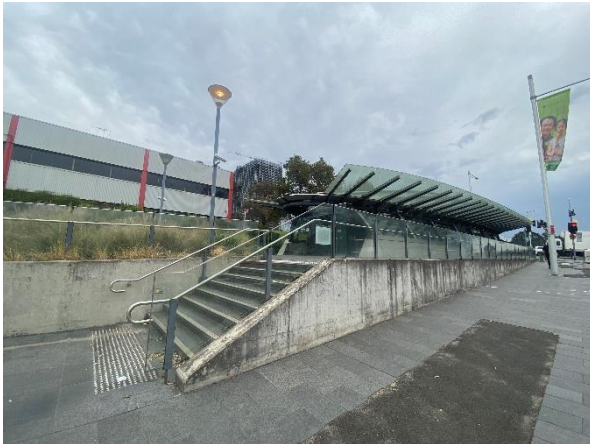
Figure 4 – The exterior of the subject site as viewed from Waterloo Road, looking south.
