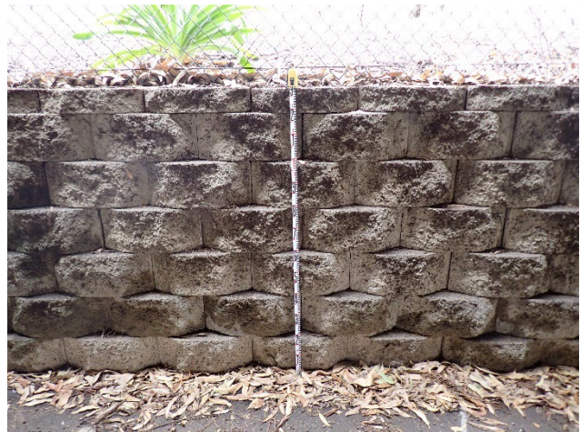
Figure 24 – Difference in level relative to south-western portion of subject area.
