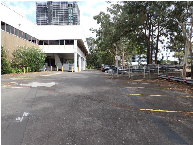
Figure 27 – Hardstand to south-west of carpark, view north-west. Note footbridge connecting with carpark roof level.
