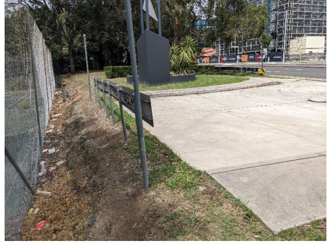
Figure 32 – North-western boundary of subject area, view south-west. Note how site steps down relative to level of Lane Cove Road.
