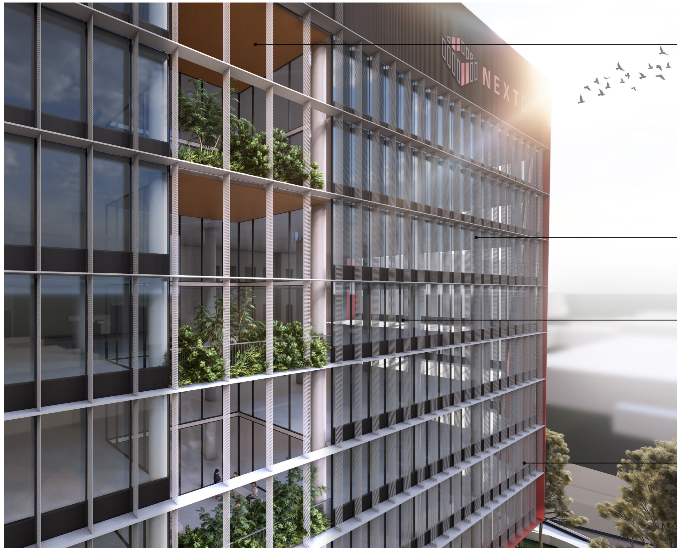
Vertical Perforated Louver Blades Poweder coated aluminium finish Color: Light grey
