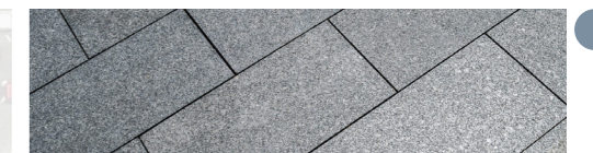
GRANITE PAVING BLACK - FLAME EXFOLIATED 600MMX300MMX60MM TO PATHS 150MMX100MMX60MM TO DRIVEWAYS
