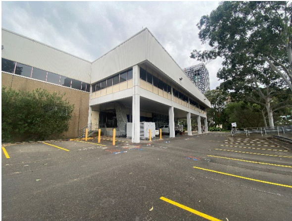
Figure 8 – Views towards warehouse 2 from within the subject site, looking southwest.
