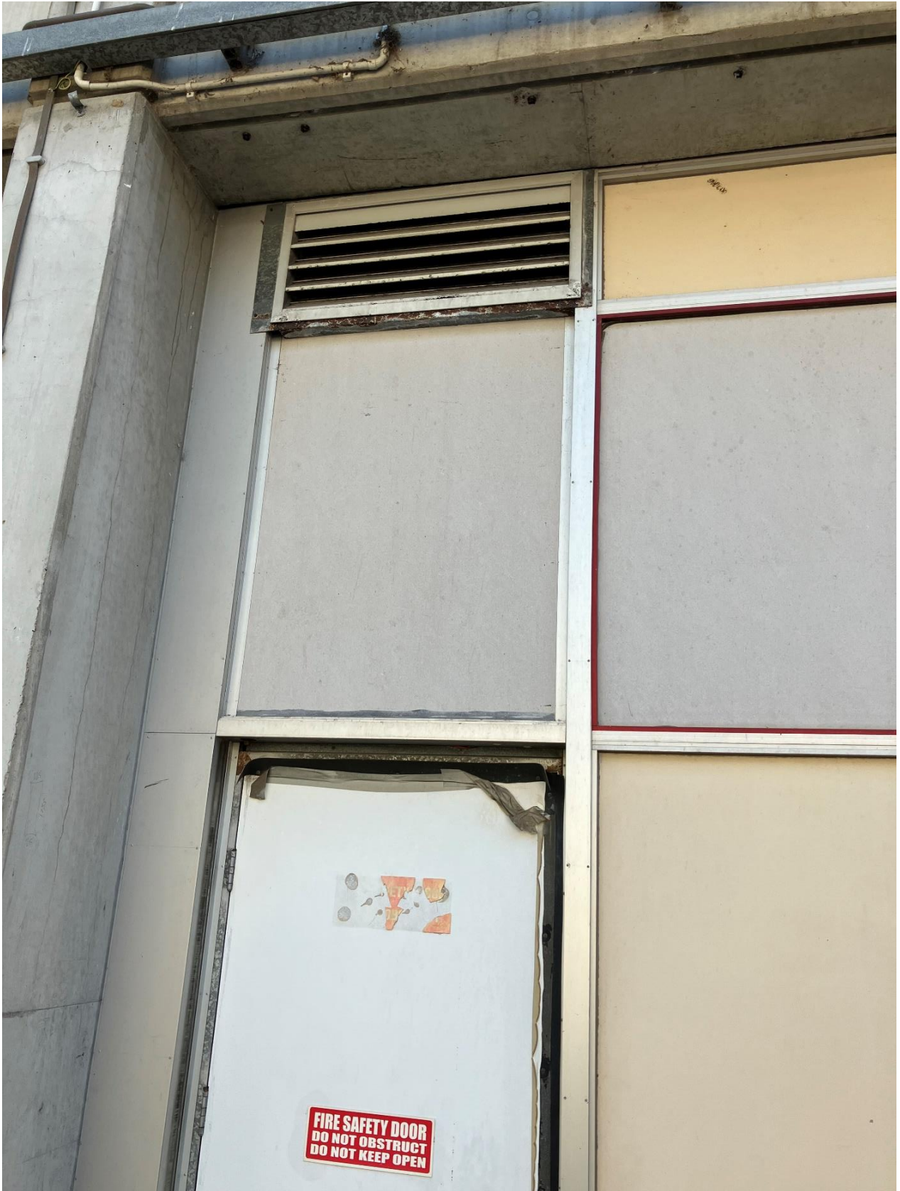
Figure 6: External air vent above fire safety door on southern building.
