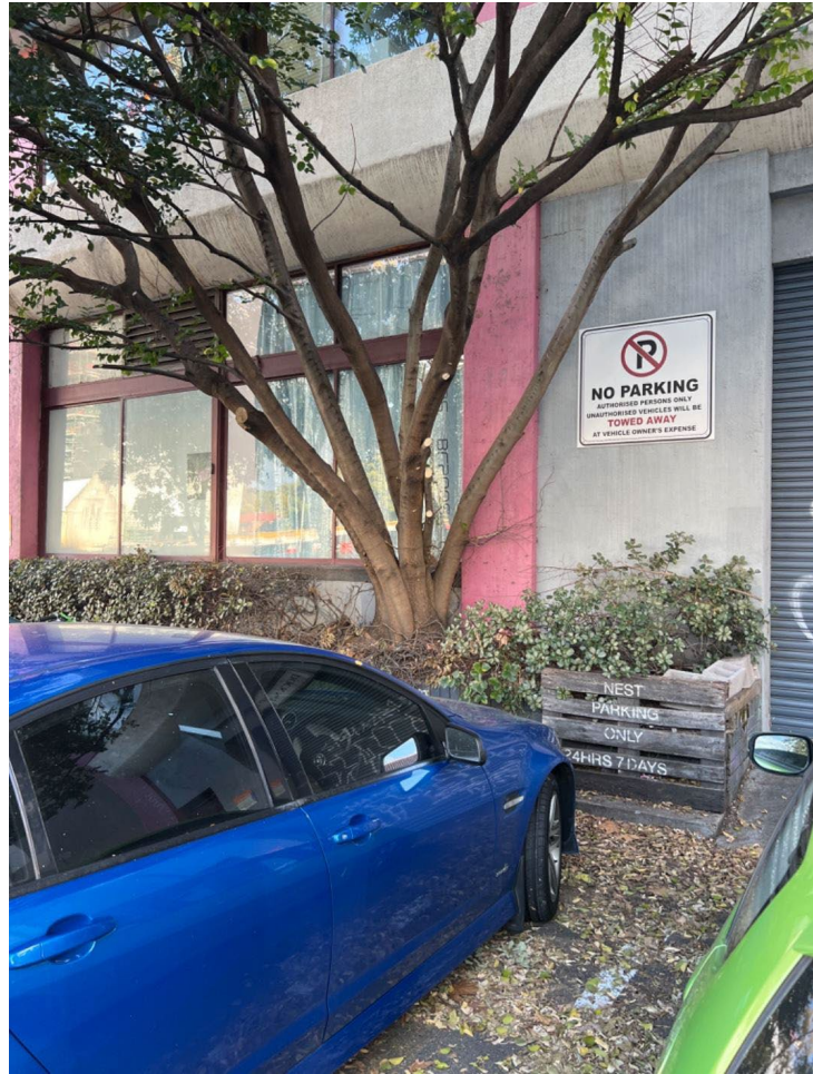
Figure 3 - Tree 2 immediately adjacent building
