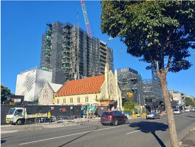
Figure 7 Adjacent future development overlooking the site
