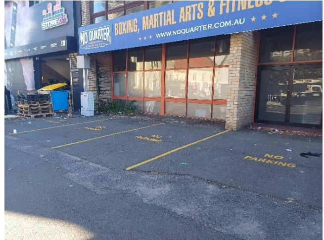
Figure 8 General carparking condition on site
