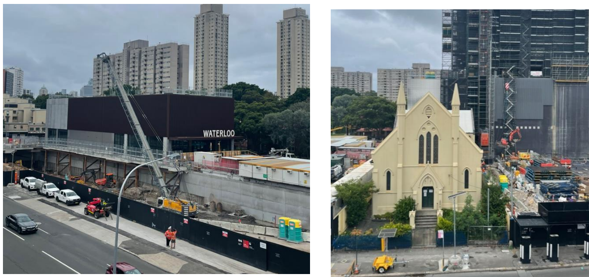
Figure 6 Waterloo Metro Station under Construction and Waterloo Congregational Church
