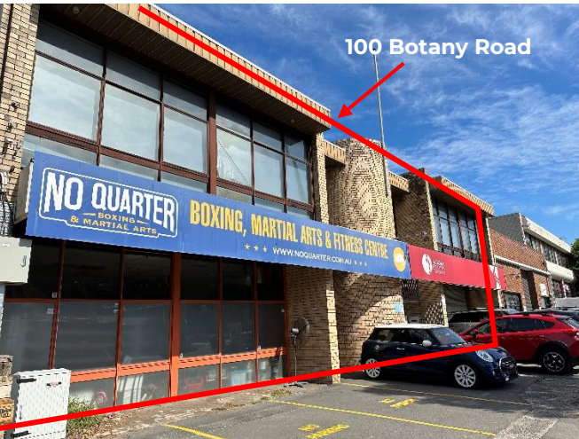
Botany Road frontage looking north.
