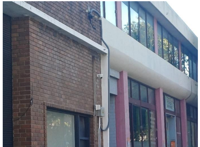
Figure 12 CCTV devices available on site
