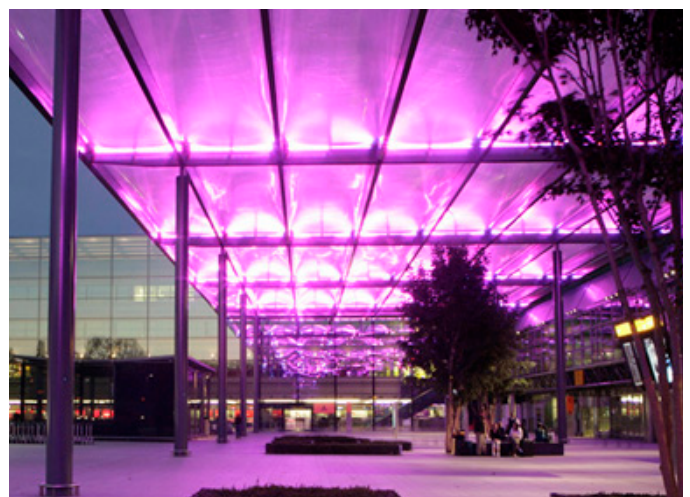
Terminal 3 Loggia, Heathrow Airport, London
