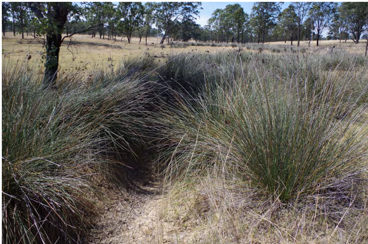
Chainage 11729 Looking Upstream
