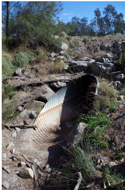
Culvert Outlet Chainage 8652 : Looking Upstream
