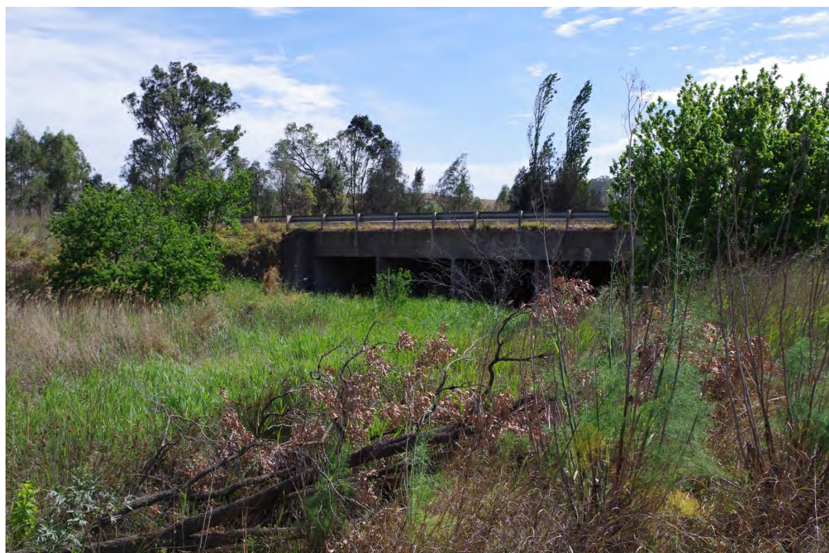
Chainage 9755 : Looking Upstream
