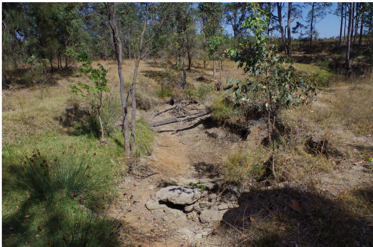
Chainage 10054 Looking Downstream
