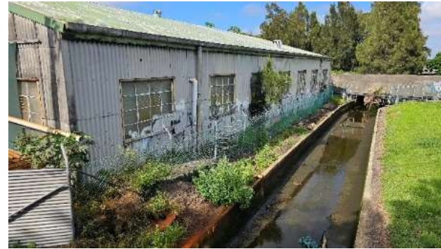
Figure 3. Current site conditions, north of the existing building, showing existing downpipe connections (to be removed).
