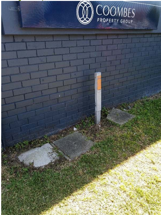
Figure 15: Services on southern boundary of study area, view to north
