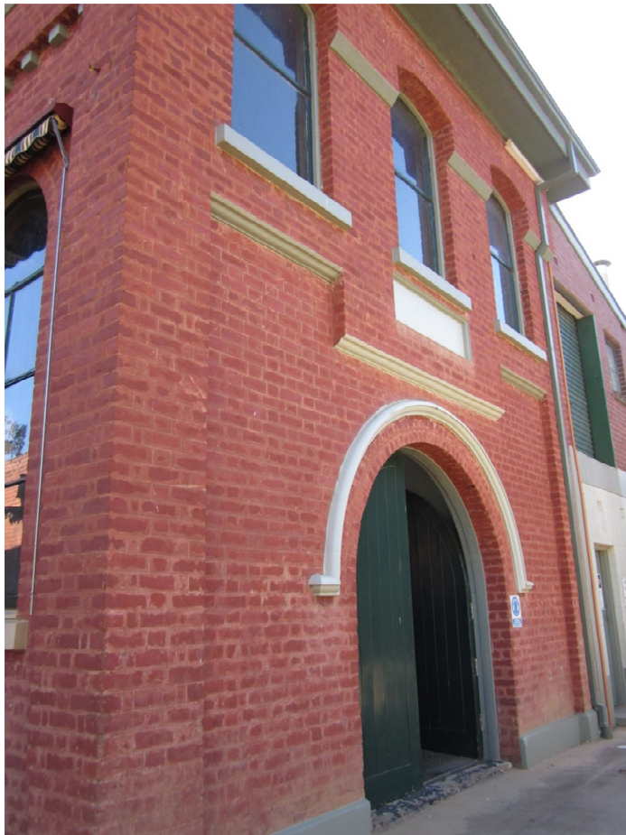
Plate 2 – Original Pumphouse Building
