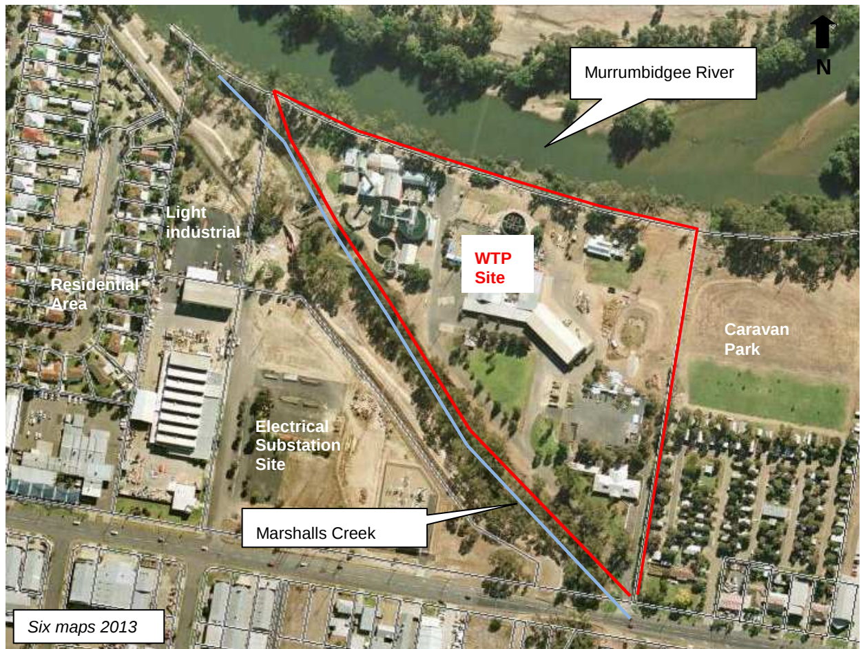
Figure 1-3 Aerial Photo of Wagga Wagga WTP and surrounding landuses
