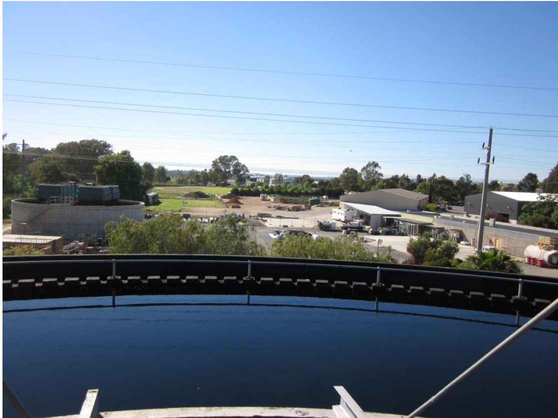
Plate 6 Showing aeration plant and builders workshop
