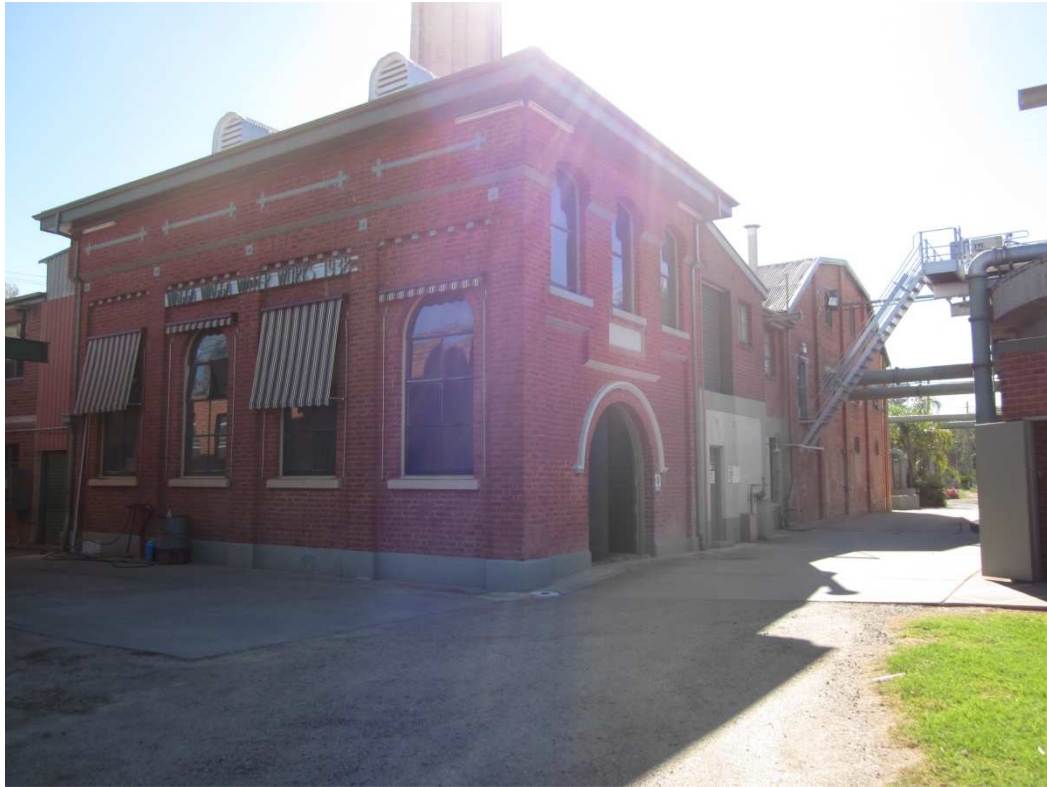
Plate 1 – Original Pumphouse Building
