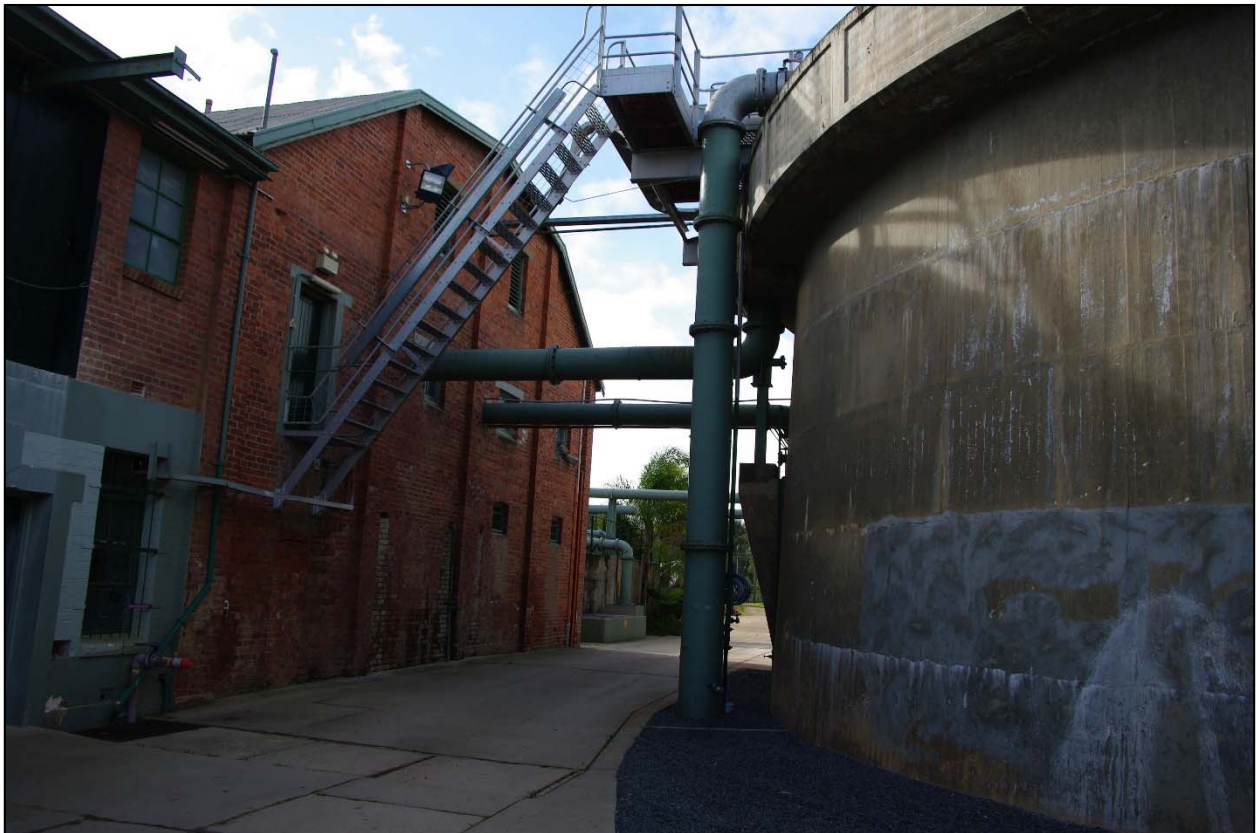
Photo 14: 1920s Boiler House (left)
