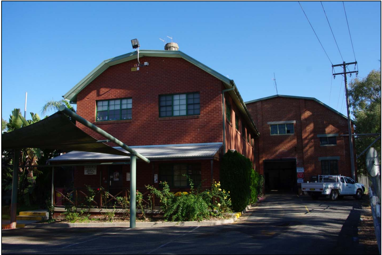
Photo 13: 1930s Workshop, right side of the image at the rear
