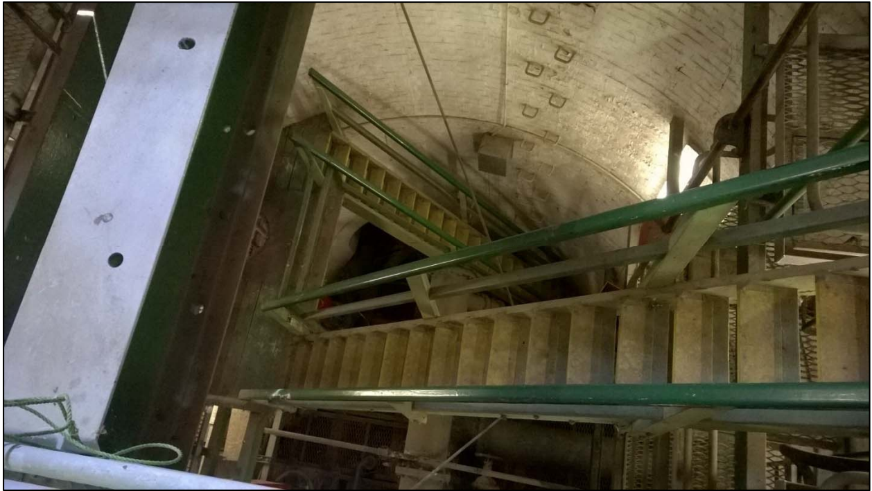
Photo 15: Brick water well
