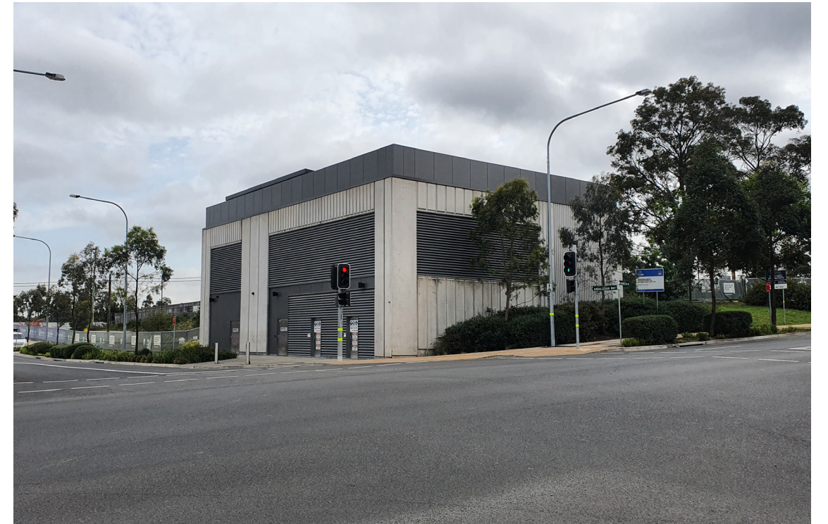
2. Metro infrastructure building to be retained, situated adjacent to the southern site's west.
