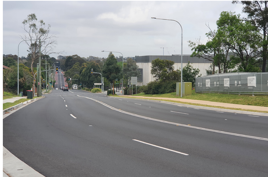
1. Carrington Road interface with the site's south continues towards Castle Hill industrial/commercial precinct.
