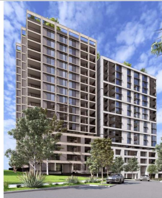
Figure 19: Northern facade of Building C (Source: Group GSA)
