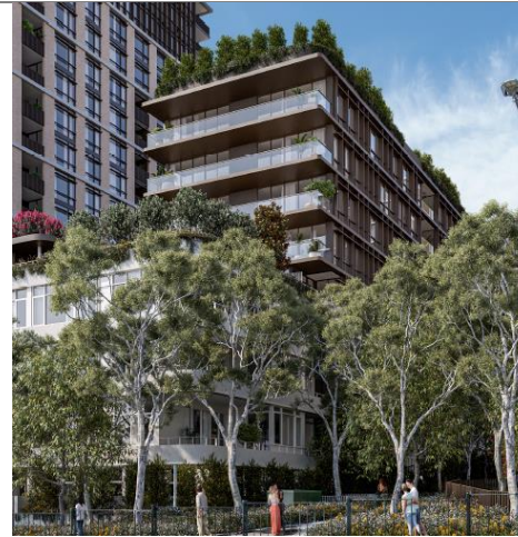
Figure 28: CGI of Building E1 from Showground Road (Source: Ivolve Studios)
