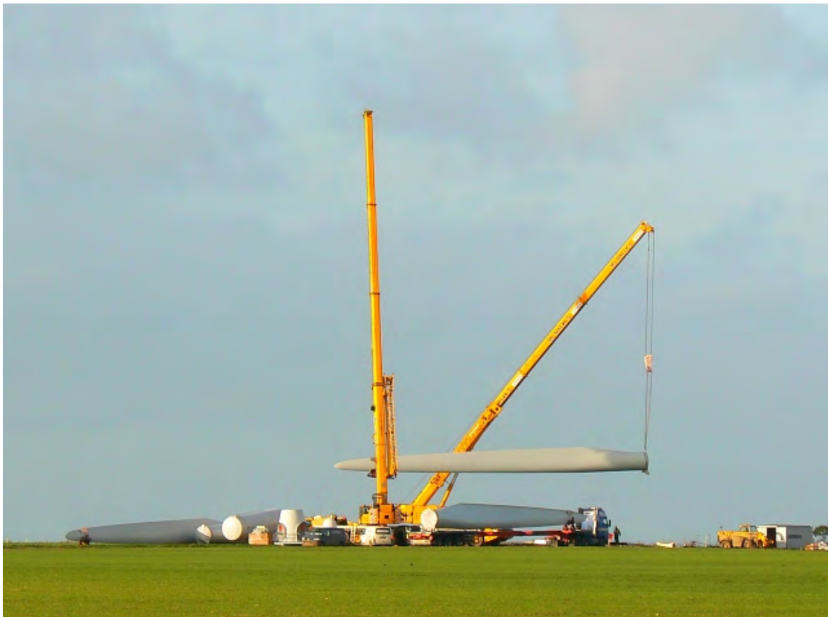
Image 4.3 - Typical WTG construction - Source: www.poweng.net
