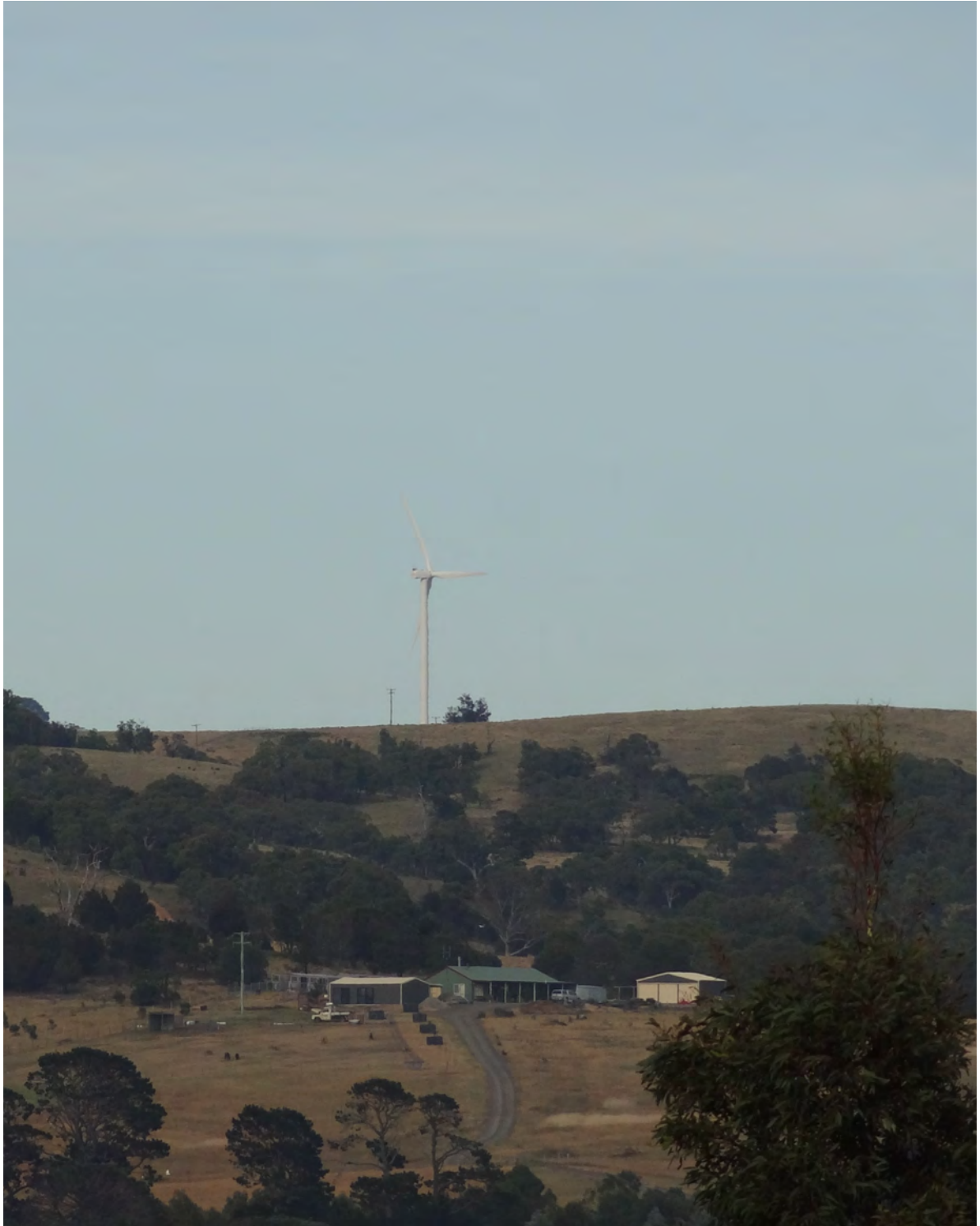
Image 5.4 -Zoomed view of Woodlawn wind farm from Lumley Road, looking west towards Tarago
