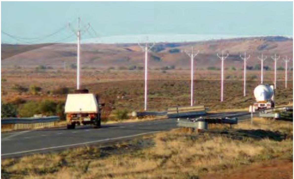
Image 4.2 - Example of similar transmission line poles alongside a road corridor - Source: https://www.ausgrid.com.au/
