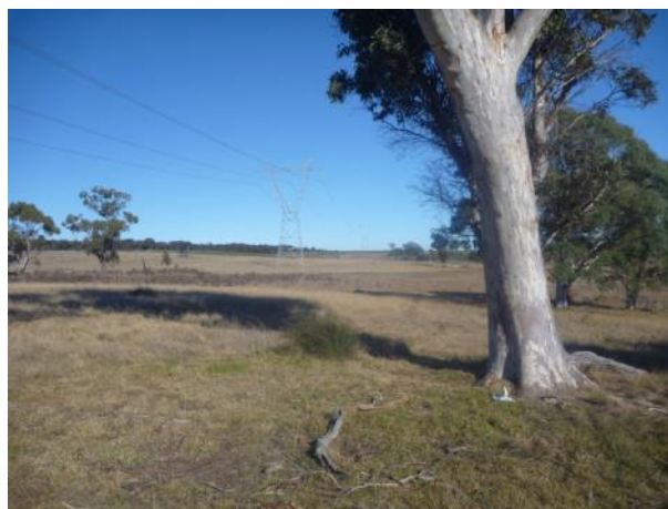
Photograph 7.46 View of JWF3 looking west (ERM 2015).
