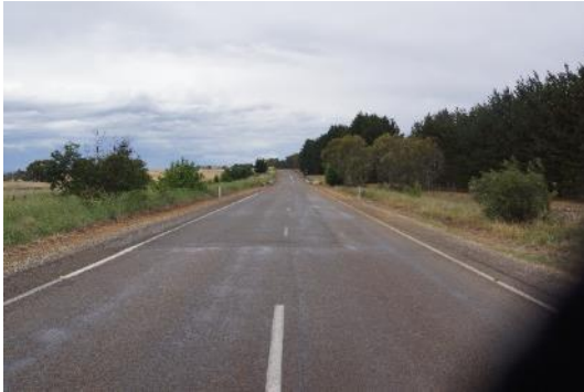
Figure 2.3: Braidwood-Goulburn Road (northern end)
