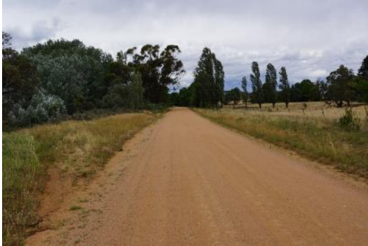
Figure 2.7: Lower Boro Road – Looking East
