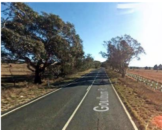
Figure 4.8: Goulburn-Braidwood Road (Northern Access 2) – Looking North
