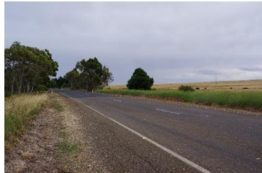
Figure 4.7: Goulburn-Braidwood Road (Northern Access 1) – Looking South
