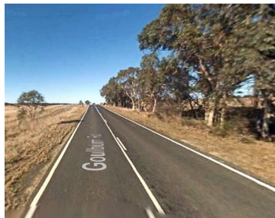
Figure 4.9: Goulburn-Braidwood Road (Northern Access 2) – Looking South
