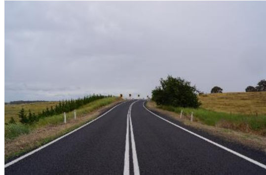
Figure 2.4: Braidwood- Goulburn Road (southern end)
