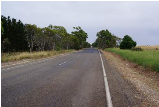
Figure 4.6: Goulburn-Braidwood Road (Northern Access 1) – Looking North
