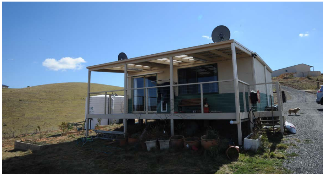
Existing dwelling – Southern façade
