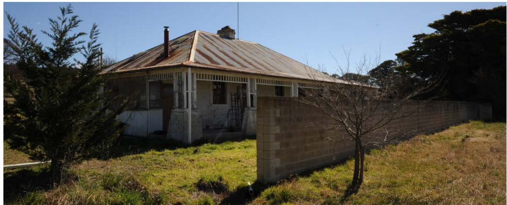
Existing Dwelling - Eastern Facade
