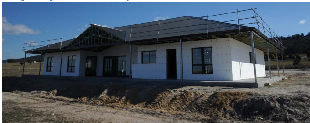
Existing Dwelling – Southern and Eastern facades
