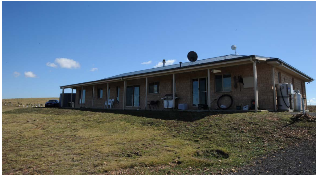
Existing dwelling – Southern façade
