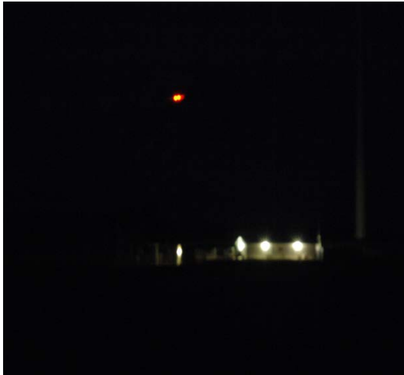
Figure 12.6 Lighting on the substation and a turbine in the background
