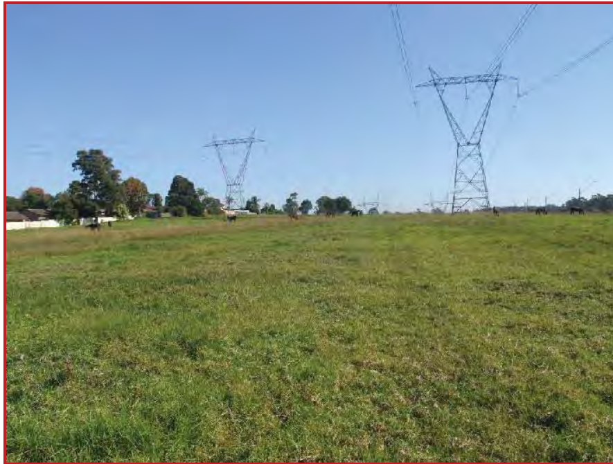
Figure 27. The transmission line forming the southern portion of the subject area, looking west.
