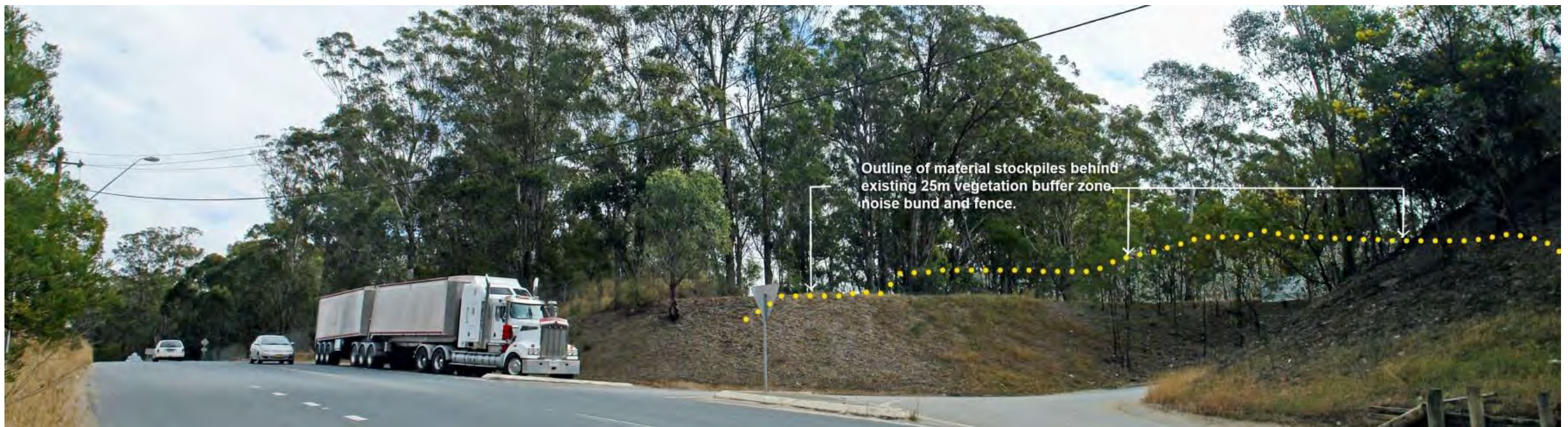
Outline of material stockpiles behind existing 25m vegetation buffer zone, noise bund and fence
