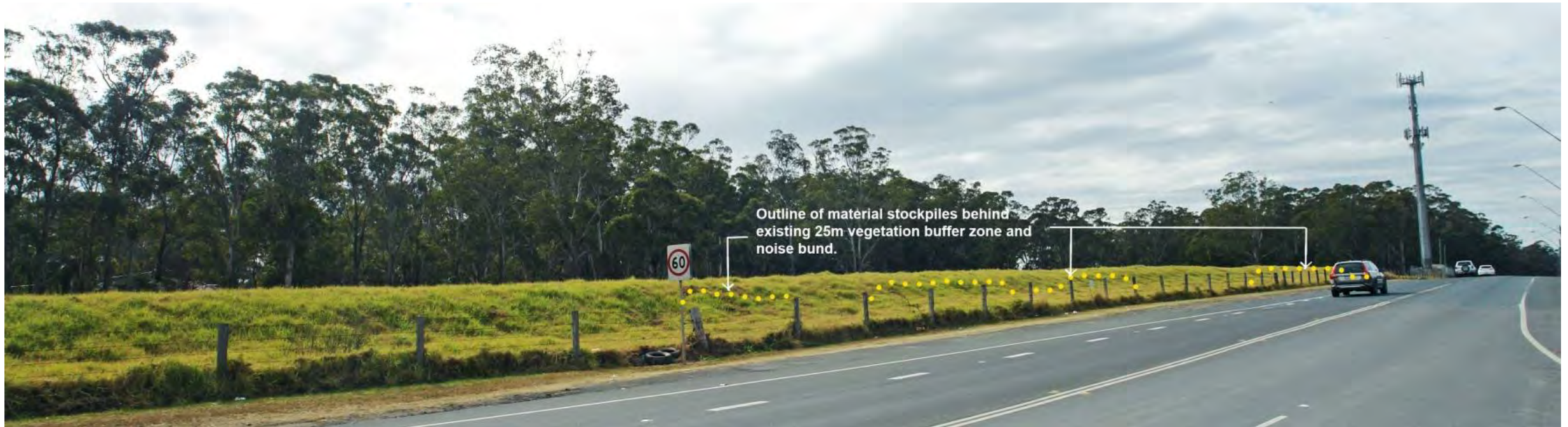
Outline of material stockpiles behind existing 25m vegetation buffer zone and noise bund
