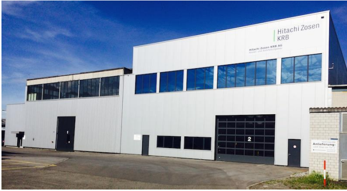
Fig. 5.5 – KRB Boiler and Piping Fabrication Workshop, HZI's wholly owned subsidiary in Buchs, Switzerland, specializing in the manufacture and repair of boiler pressure parts and equipment components (KRB)
