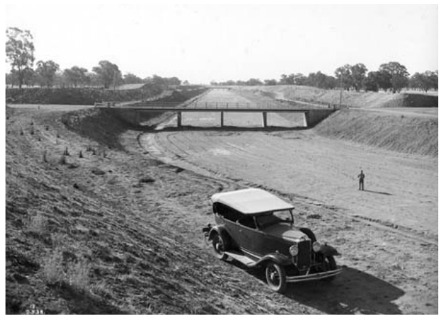
Figure 13 – Construction of the Mulwala Canal, showing the depth and extent of ground disturbance. Source: State Water Archives Collection.
