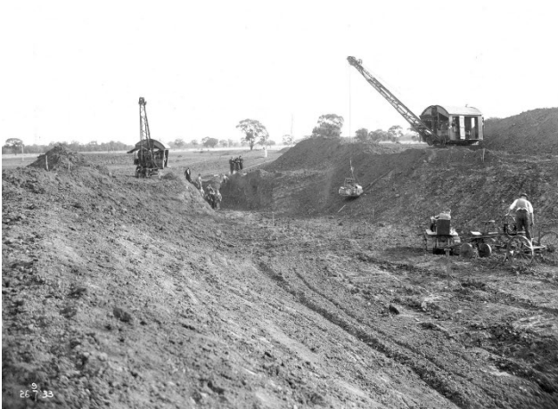
Figure 12 – Construction of the Mulwala Canal using Bucyrus Erie dragline excavators. Source: State Water Archives Collection.
