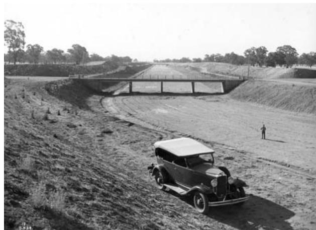
Figure 12 – Construction of the Mulwala Canal, showing the depth and extent of ground disturbance. Source: State Water Archives Collection.
