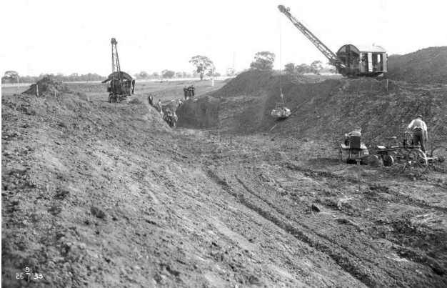
Figure 11 – Construction of the Mulwala Canal using Bucyrus Erie dragline excavators. Source: State Water Archives Collection.
