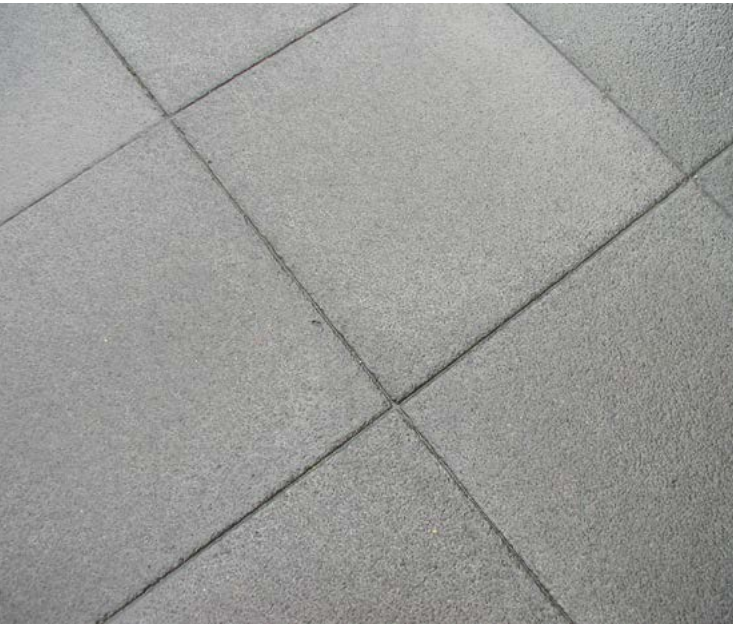
CONCRETE UNIT PAVERS TO BUILDING FORECOURT
