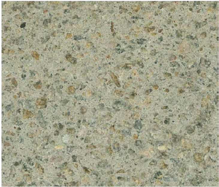
FORMAL EXPOSED AGGREGATE CONCRETE FOOTPATH
