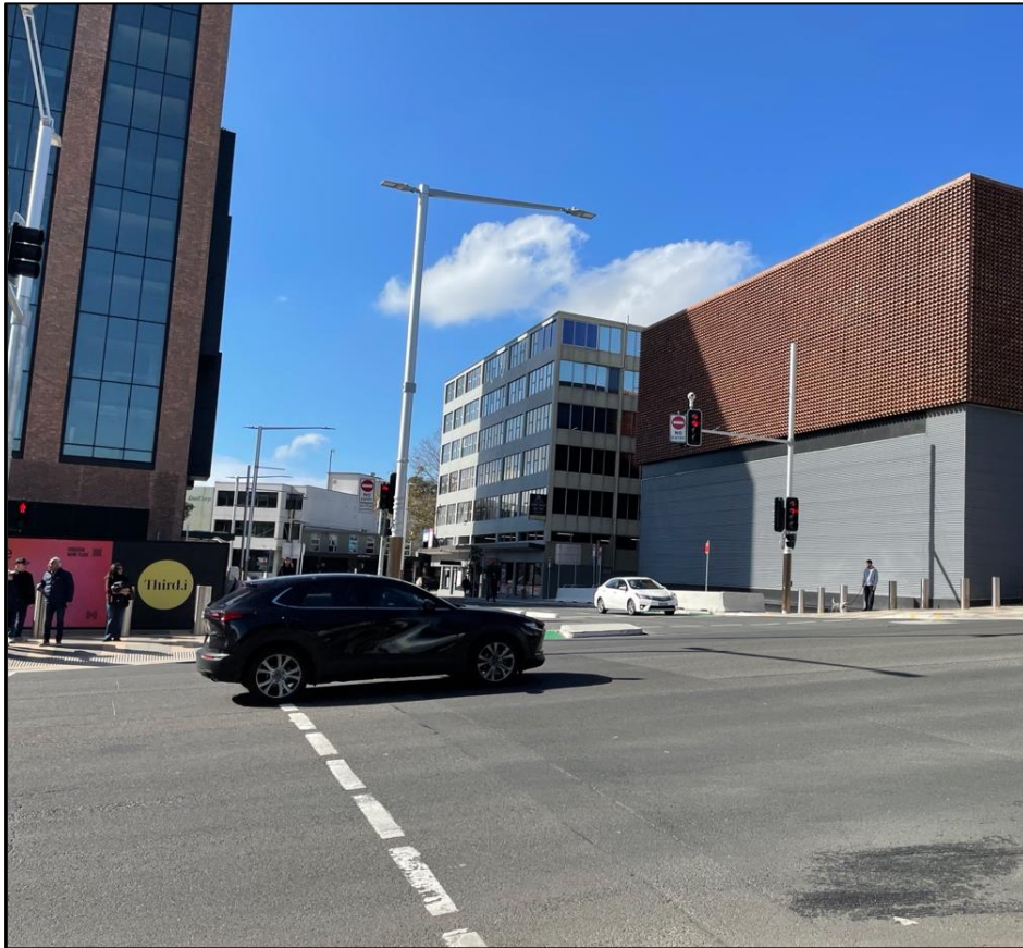
Figure 6. View from the corner of Hume Street and Pacific Highway looking East to Site B (July 2025)
