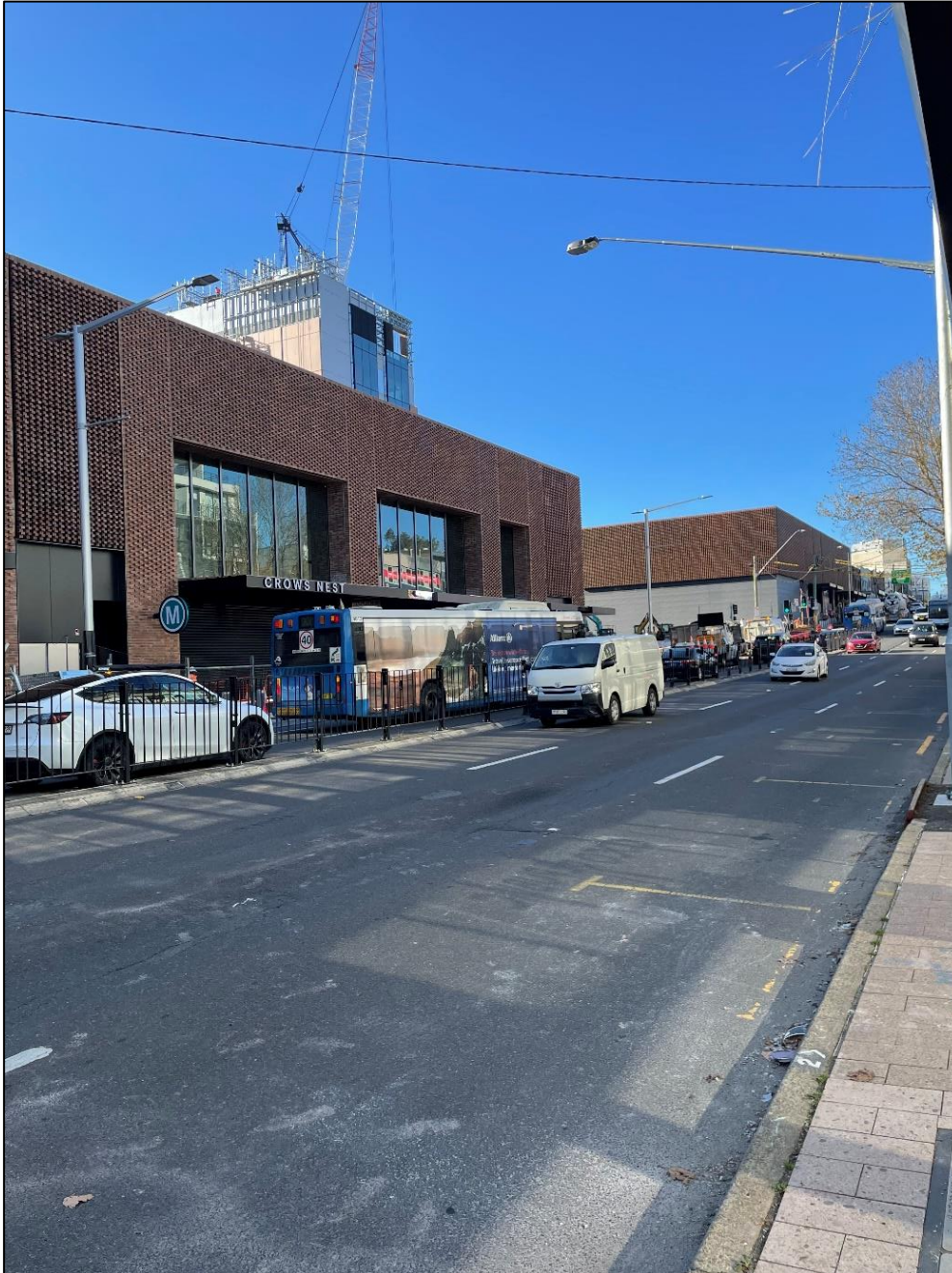
Figure 4. View from Pacific Highway looking South to Site B (July 2024)
