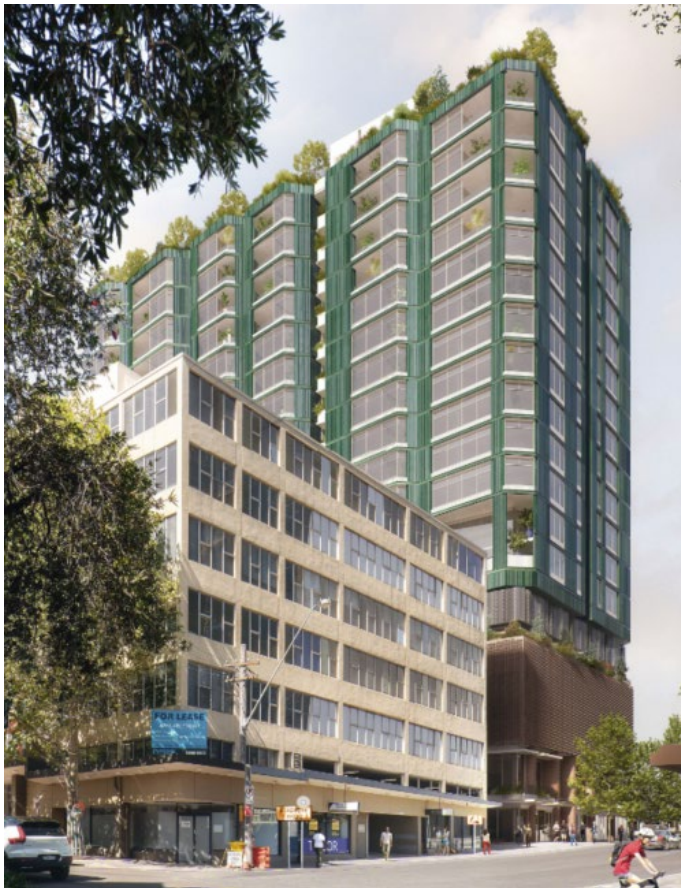
Figure 4: View of the proposed development from the north, showing the Hume St and Clarke Lane elevations
