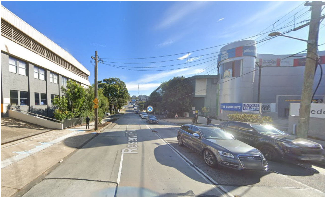
Figure 3-11: Landscape Character Zone 2 - Artarmon Industrial Estate (Photo: Google Maps)
