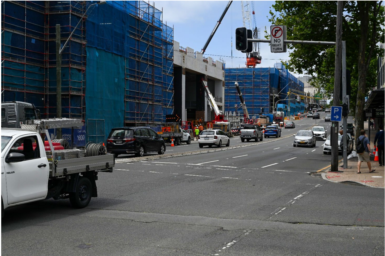
Figure 5-20 Viewpoint 10 – Oxley Street at Pacific Highway (Photo: RPS)
