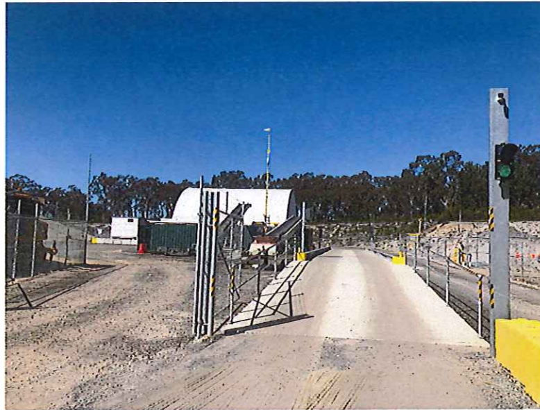
Photo 6 - Weighbridge looking south
