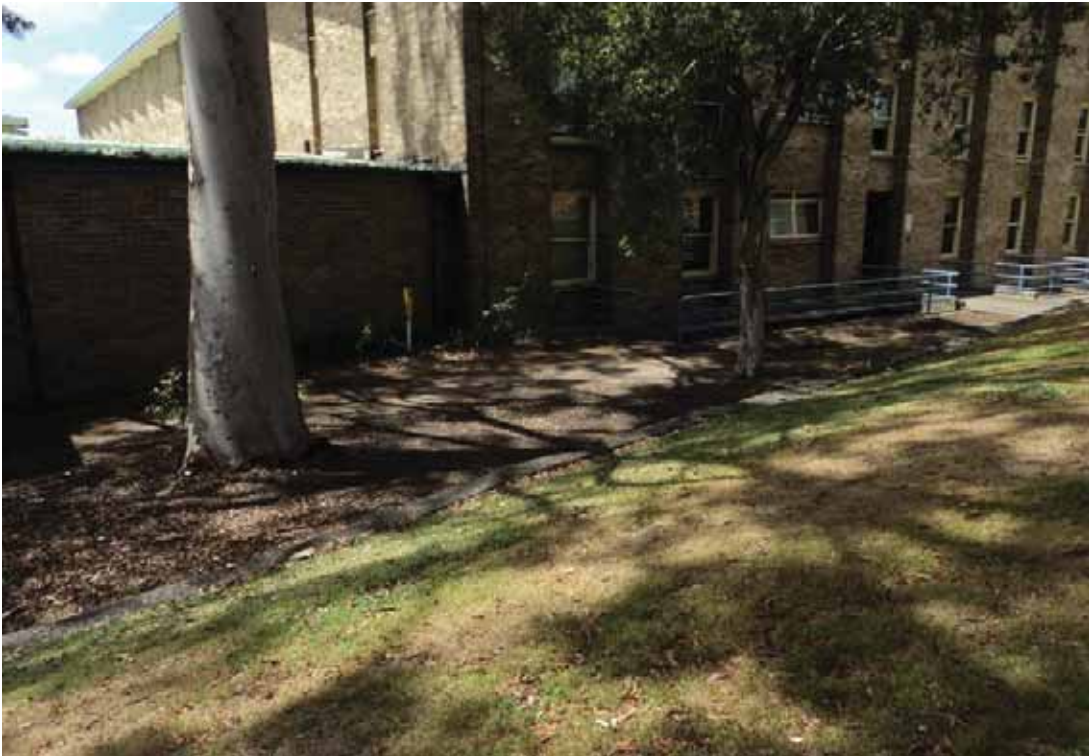
Photo 2 - Ground sloping towards Merewether Building
