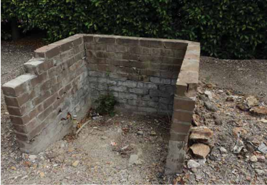
Photo 19 - Fill behind demountable buildings
