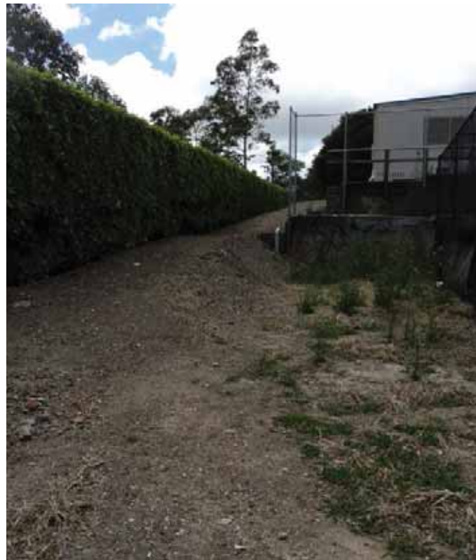
Photo 18 - Fill behind demountable Buildings
