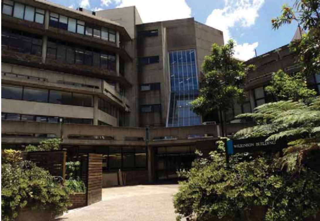
Photo 5 - Wilkinson Building facing west
