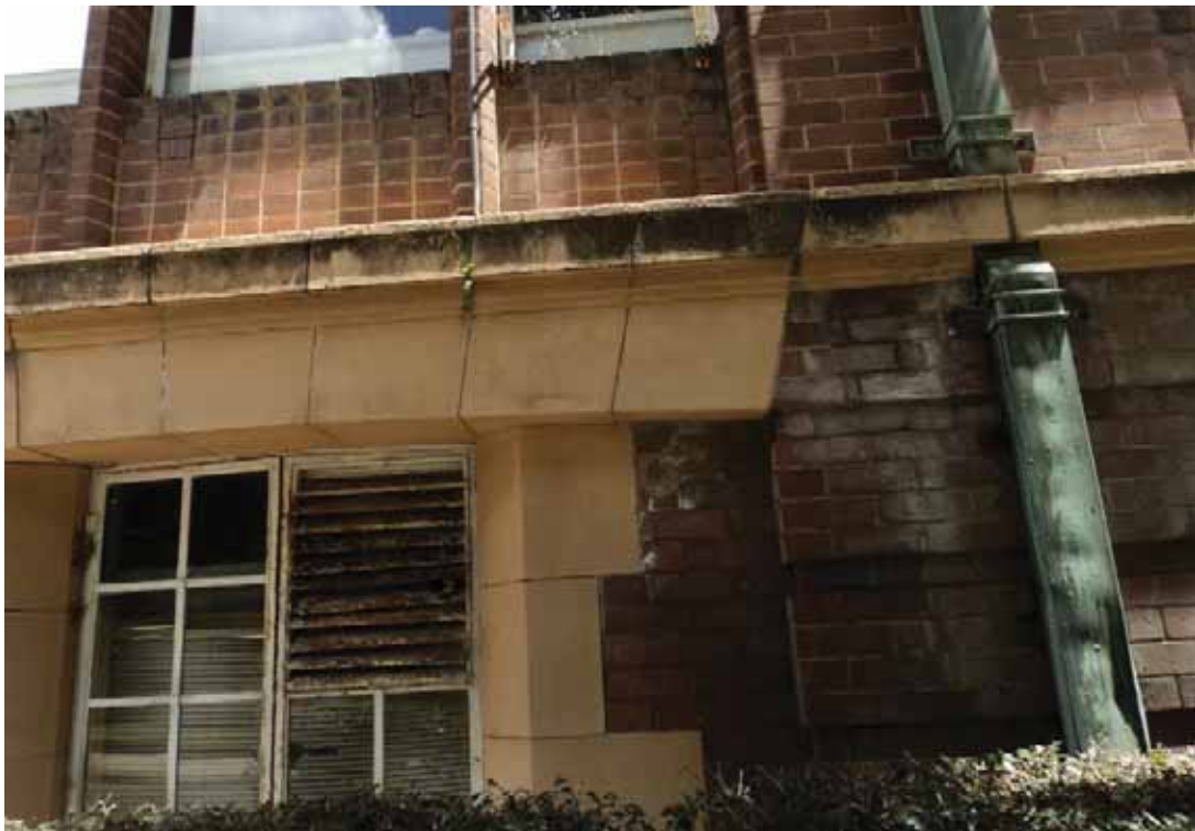
Photo 12 - External Facade Blackburn Building
