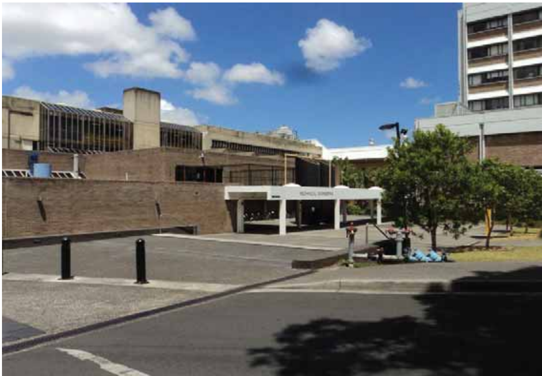
Photo 6 - Mechanical Engineering Building
