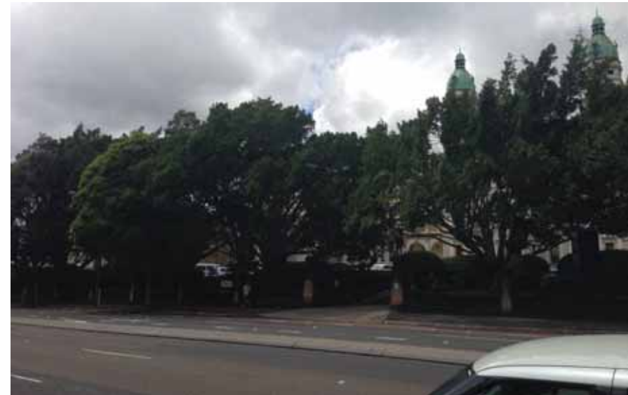
PICTURE 3 – THE INSTITUTE BUILDING BEYOND ESTABLISHED VEGETATION VIEWED FROM CITY ROAD
