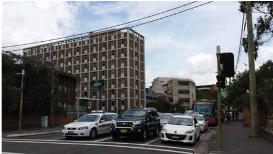
PICTURE 1 – CITY ROAD PRECINCT VIEWED FROM CITY ROAD AND AT INTERSECTION WITH CLEVELAND STREET
