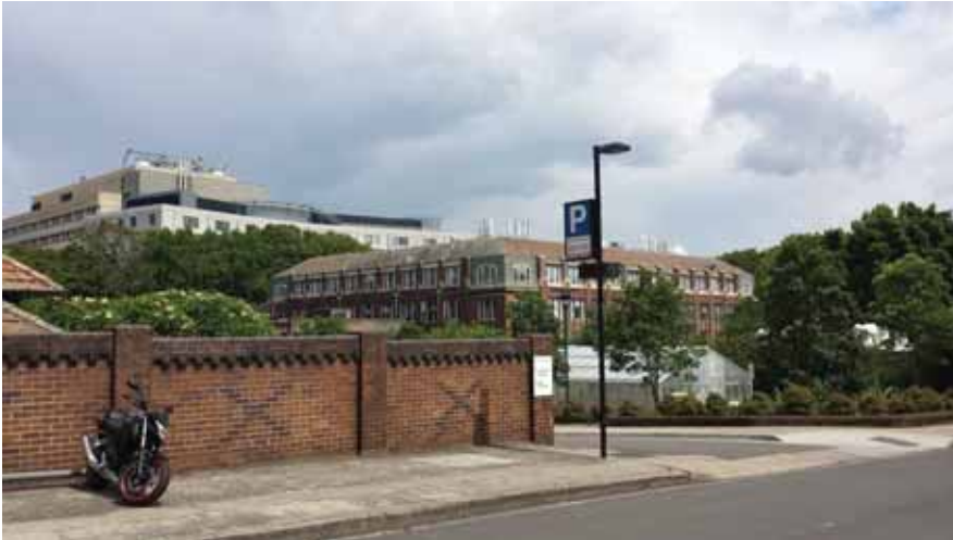
PICTURE 5 – THE BLACKBURN BUILDING AND BOSCH GLASSHOUSES (AND RPA BEHIND) VIEWED FROM THE WESTERN AVENUE AND THE HEALTH PRECINCT
