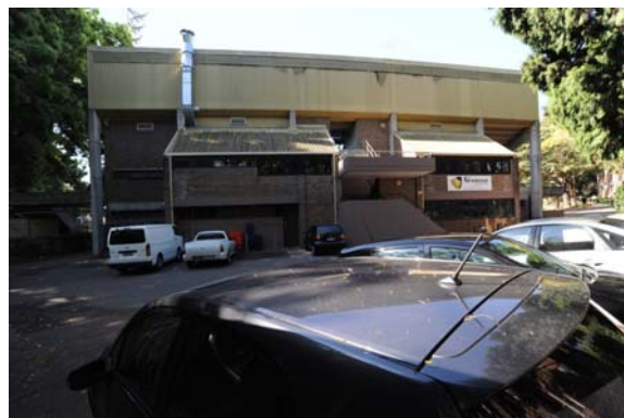
Figure 49: Rear of the Bruce Williams Pavilion
