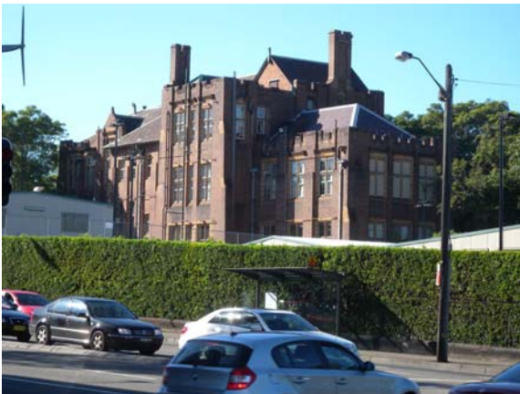
Figure 38: RD Watt building (as seen from Parramatta Road)
