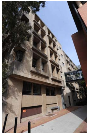
Figure 35: RMC Gunn Building
