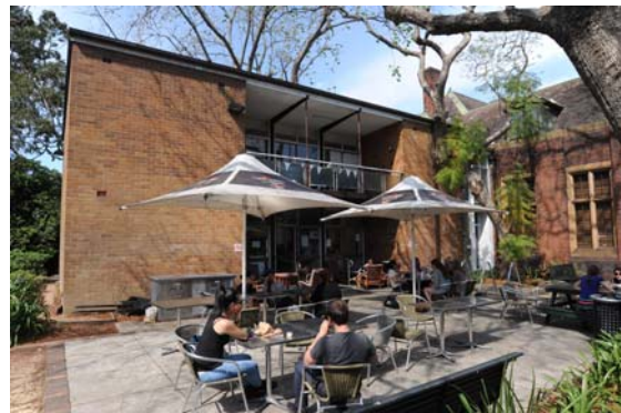
Figure 27: North wing of JD Stewart Building
